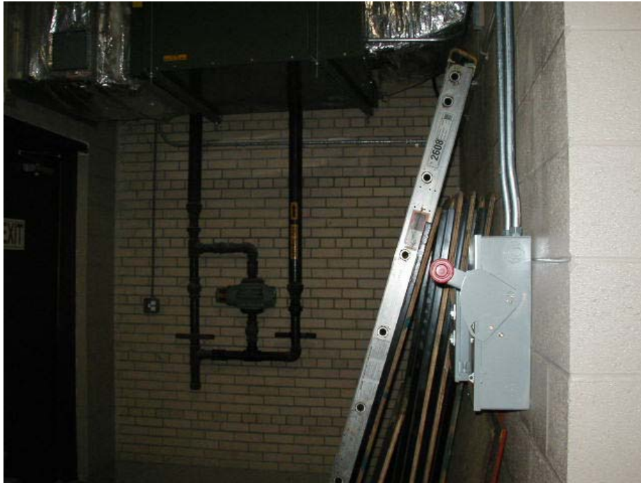
Looking west at wall that separates manufacturing area from warehouse. Wall at right is the south wall of chemical storage room. Door at left opens onto the parking lot area on the south of the warehouse
