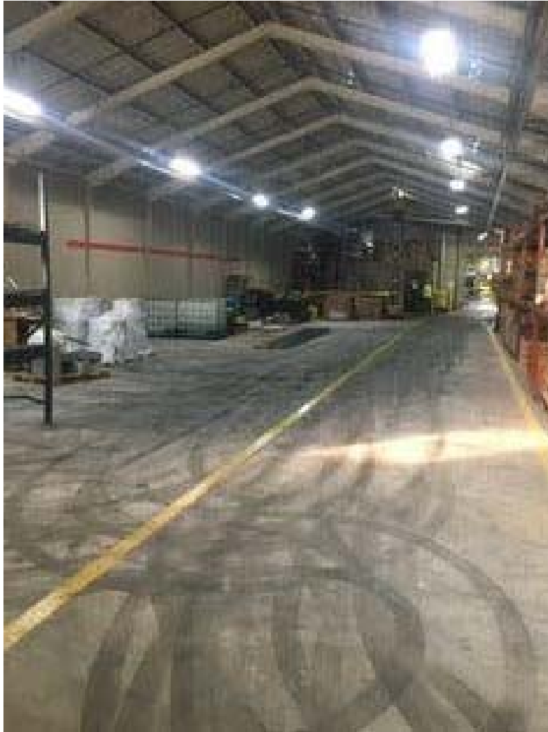
View of concrete floor on south side of warehouse, facing west.
