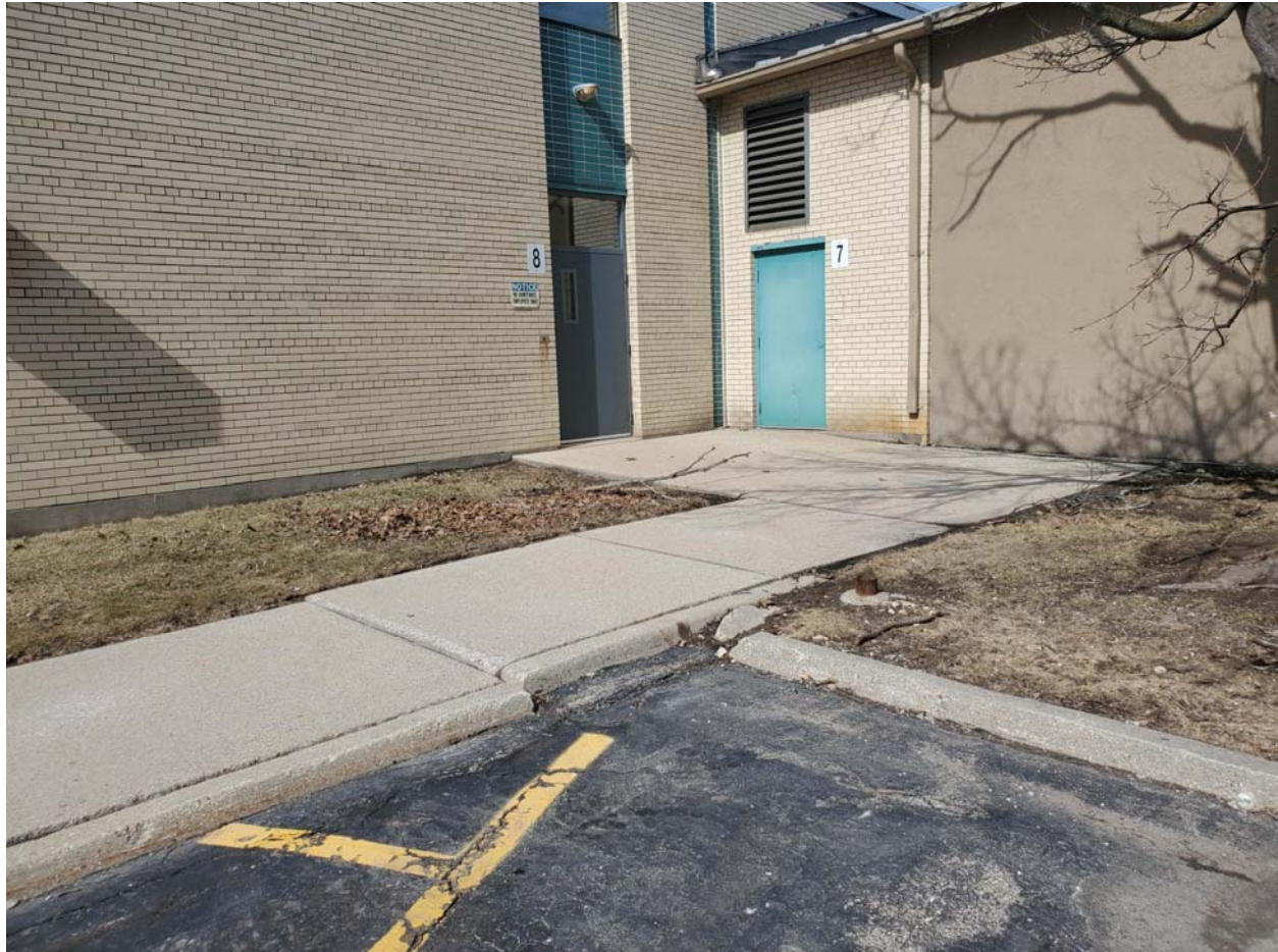
View of grass and concrete portions of the cap outside the southwest corner of the warehouse, facing northwest. The asphalt in the photo is on the 714 Hancock Street parcel.
