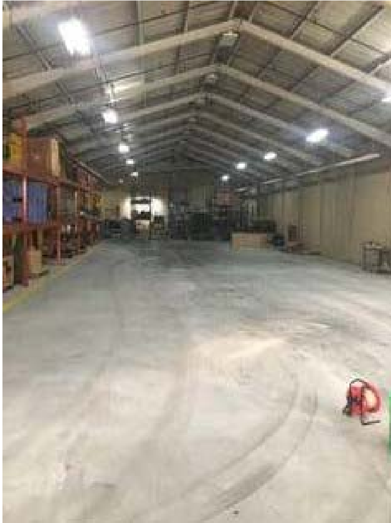
View of concrete floor on north side of warehouse, facing west.
