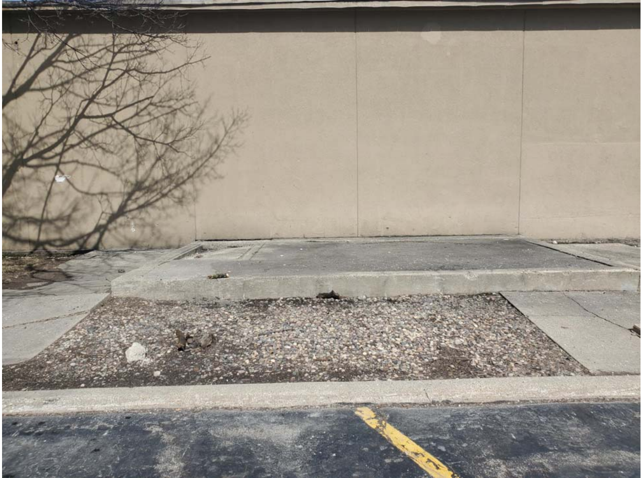
View of gravel and concrete portions of the cap, facing north.
