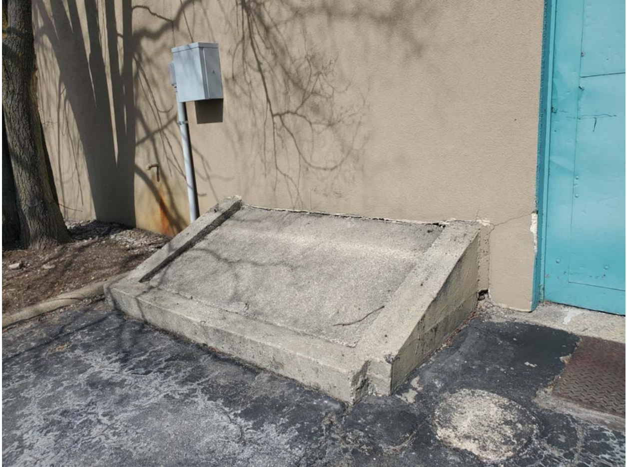
View of a concrete surface feature near the southeast corner of the warehouse, facing northwest.
