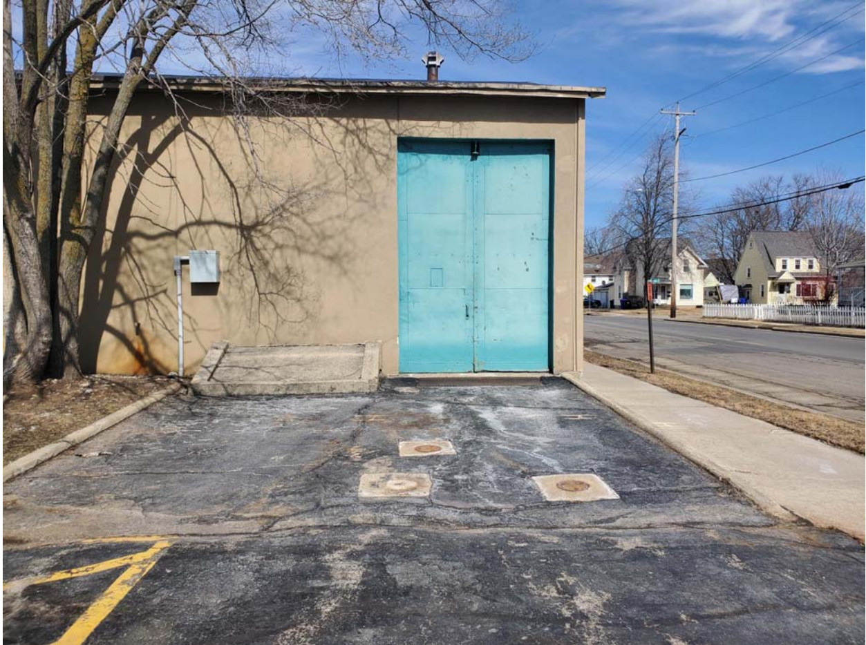
View of the asphalt portion of the cap, facing north.
