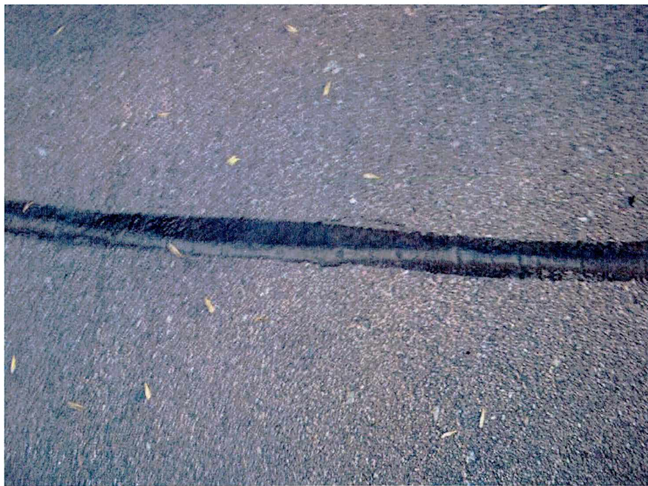
Photo 4 – Close-up of crack repair.
