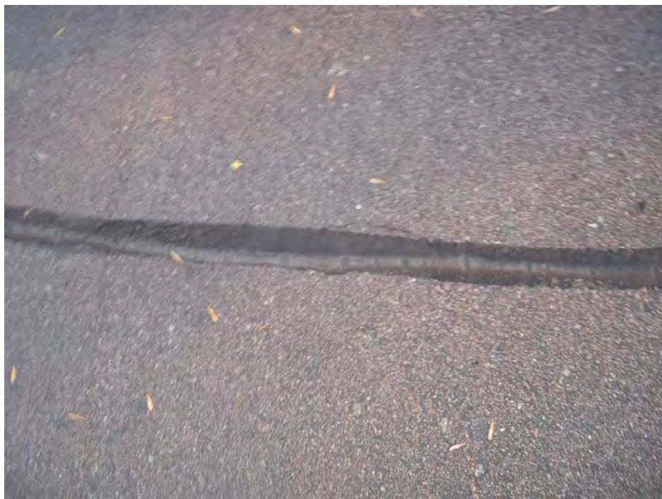
Photo 4 – Close-up of crack repair.
