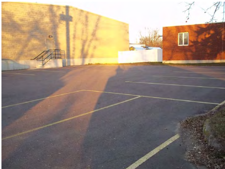
Photo 1 – Parking lot south of Wausau Chemical. Looking northeast.
