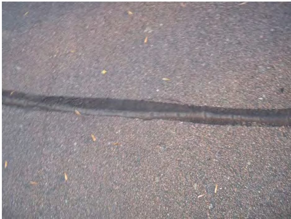
Photo 4 – Close-up of crack repair.
