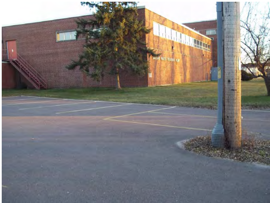
Photo 2 – Parking lot south of Wausau Chemical. Looking southeast.
