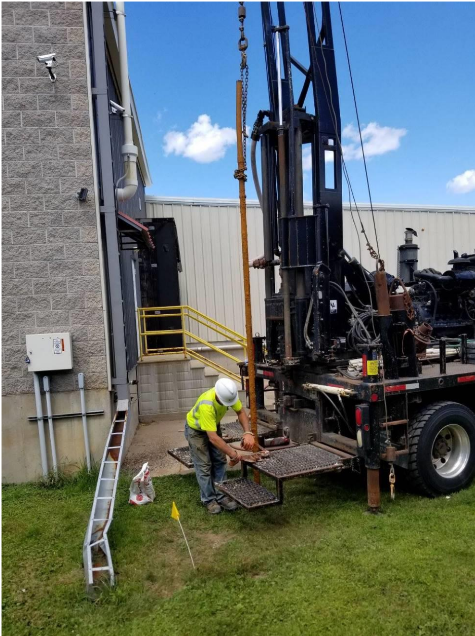
Photo 2 - CW3 casing removal
