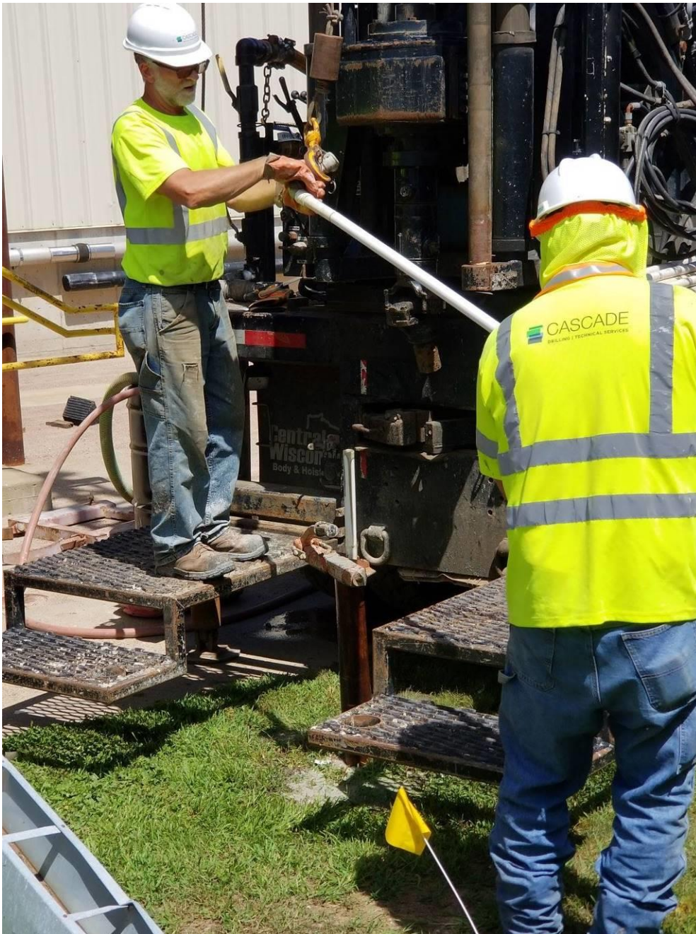
Photo 1 - CW3 grouting via tremie
