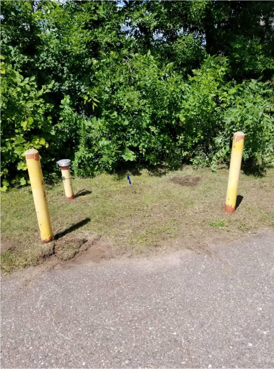
Photo 3 - CW4 after sealing (CW4A to the left)
