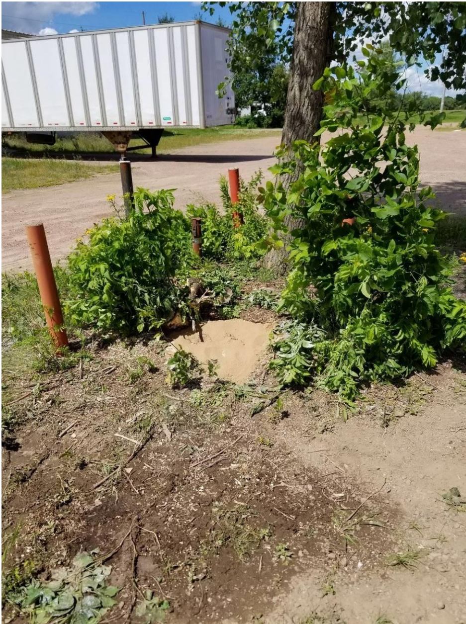
Photo 4 - CW5 after sealing (CW5A in background)
