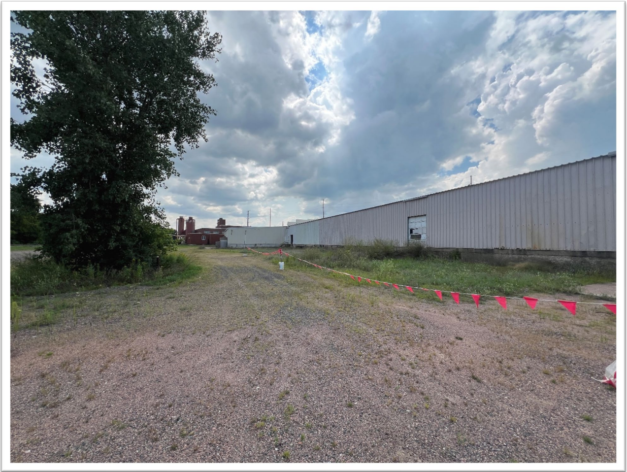
Image 5: Wausau Chemical building and MW WC5A (overgrown) on the East Bank facing south
