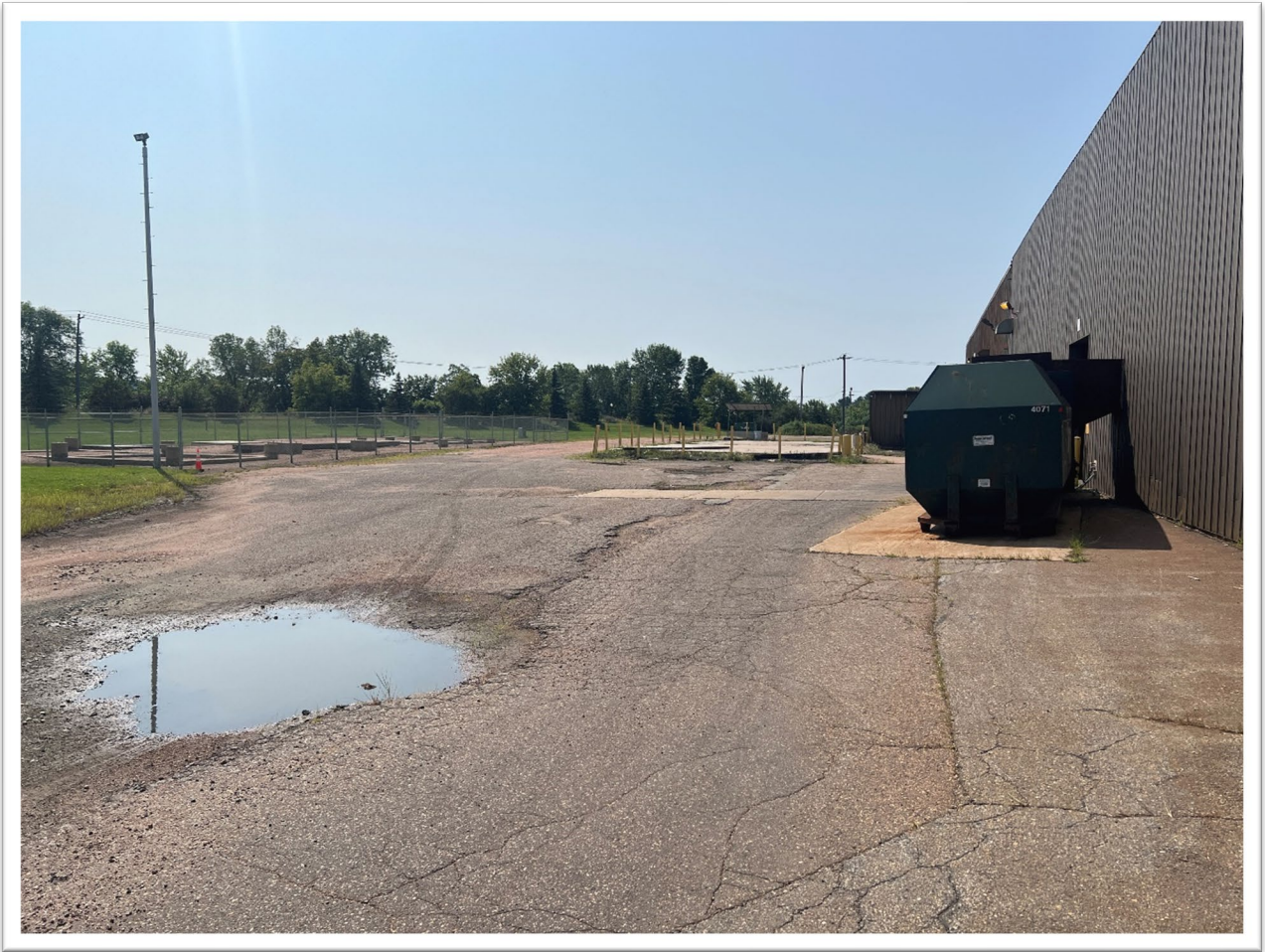
Image 4: Photo of landfill cap taken facing south
