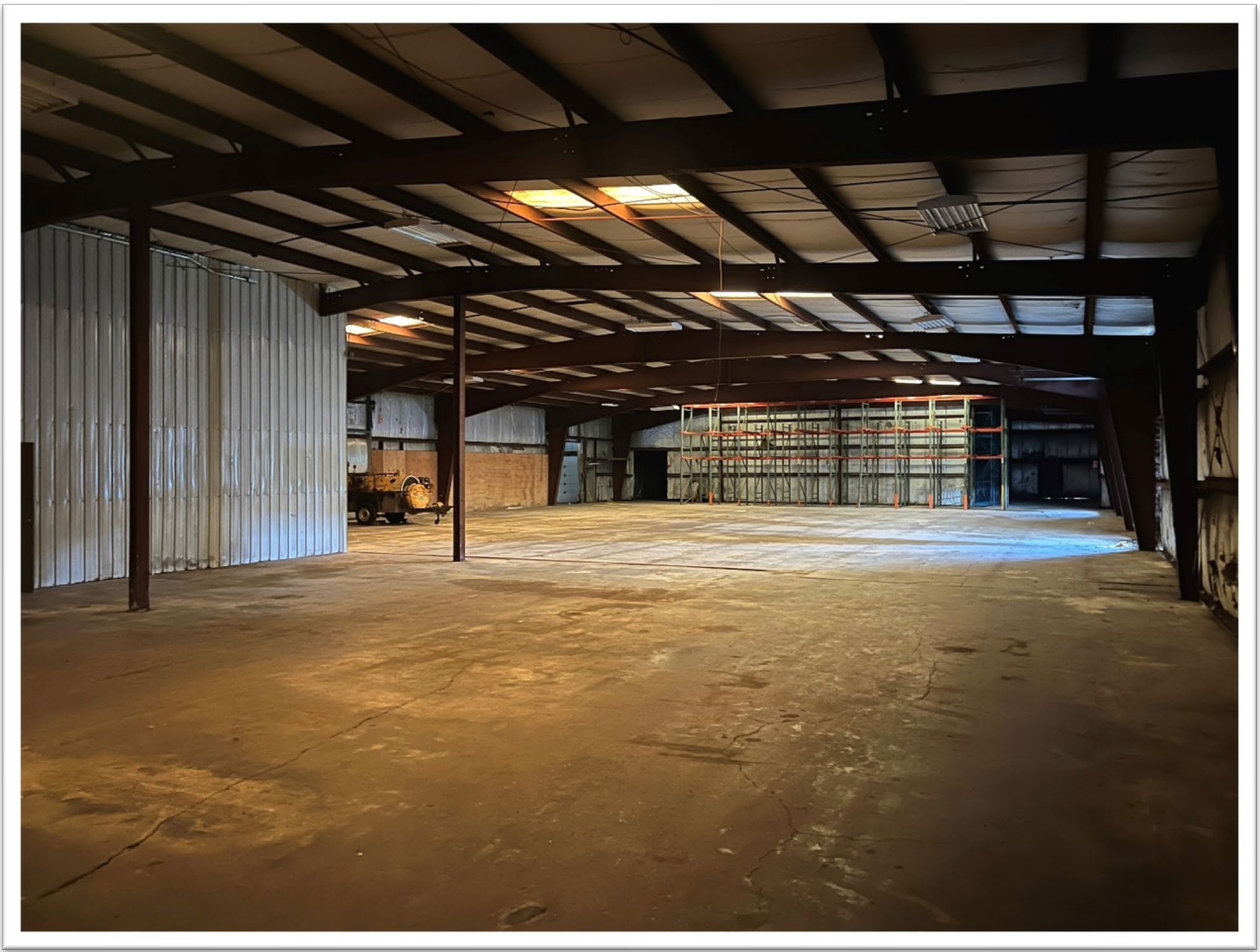
Image 6: Interior of the Wausau Chemical building showing that it is clean and maintained
