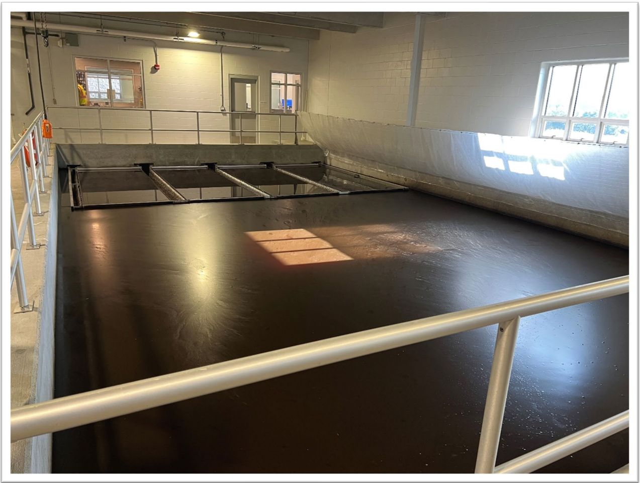
Image 1: Flocculation tank at Wausau Water Works which was recently constructed in 2022
