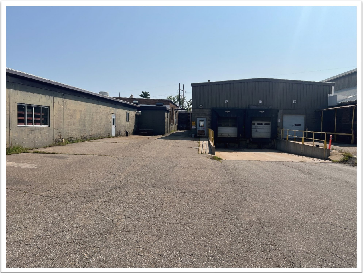
Image 8: Area north of old foundry area where drums had historically been stored
