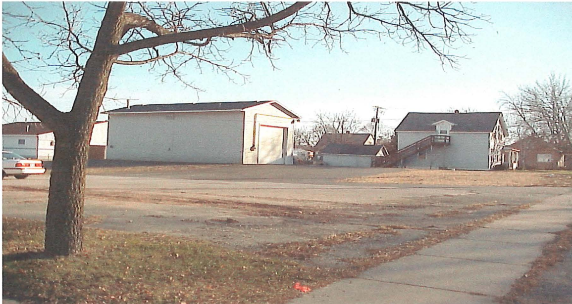
Relocated treatment building at Zinc Shop.
