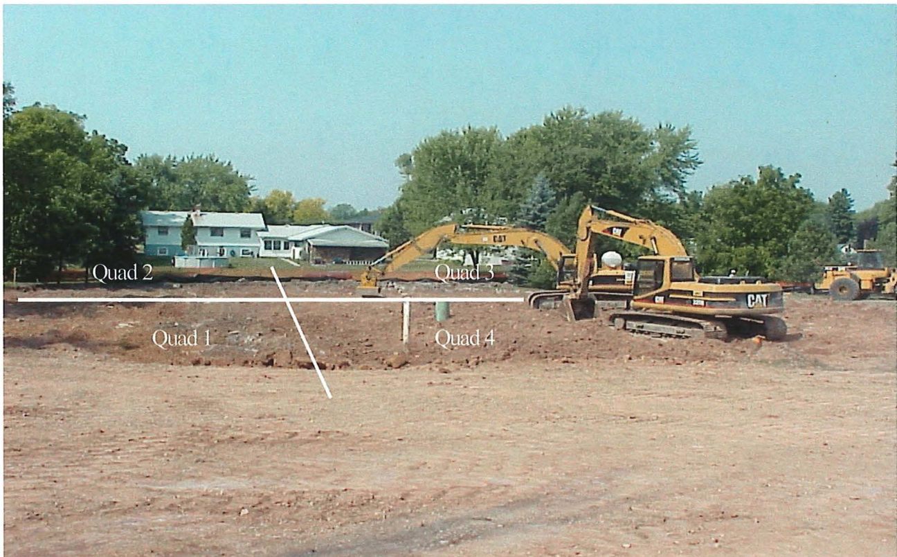
Extent of excavation at Chrome Shop Site with approximate excavation quadrants indicated
