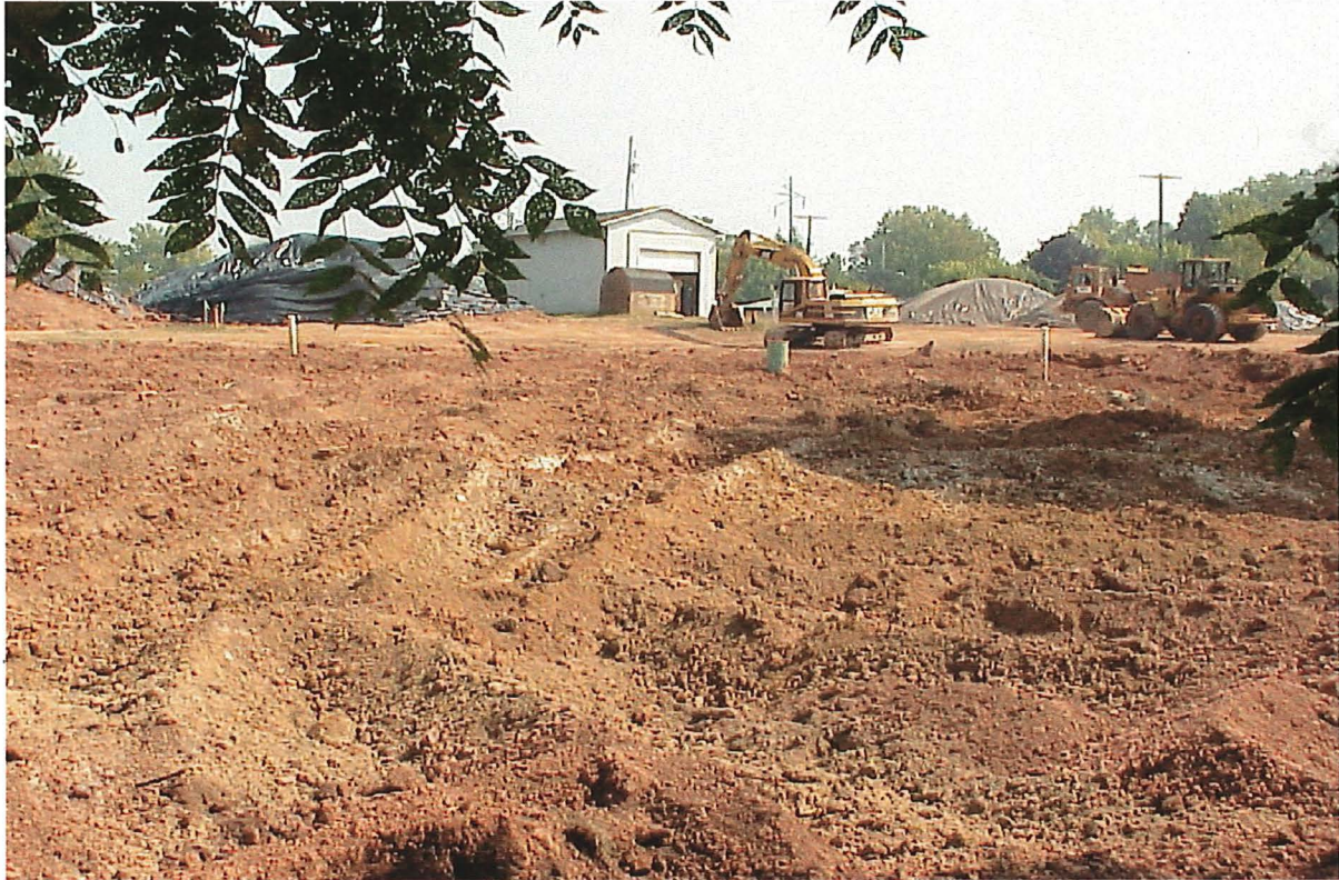
Excavated area at Chrome Shop looking northeast from southwest property corner. Treated soil in foreground (Quad. 2) prior to stockpiling.
