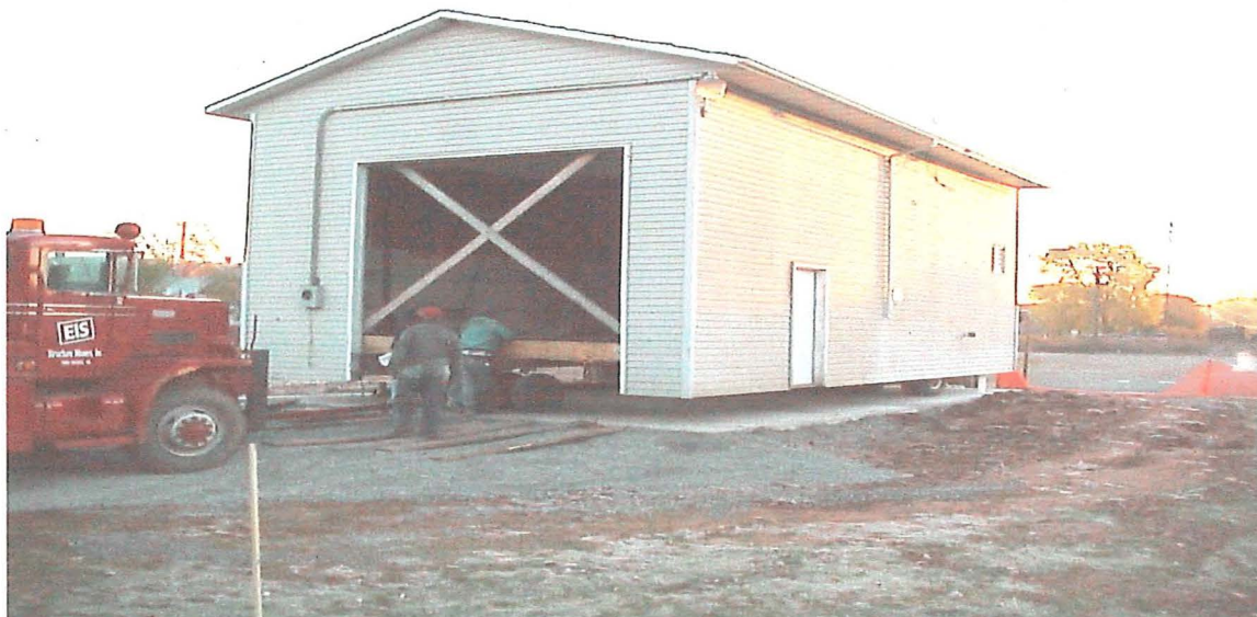
Treatment building on new slab foundation at Zinc Shop
