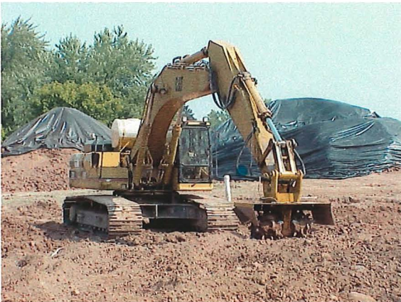
Backhoe with roto-tiller attachment
