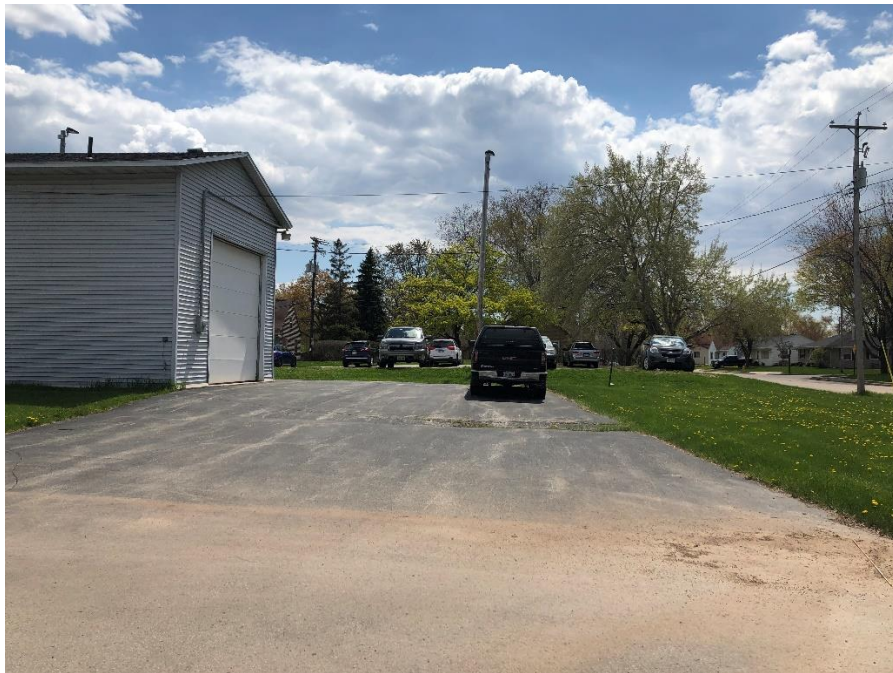
Photo 4 Description: Pump and treatment system house and additional parking lot in background Location: Zinc Shop
