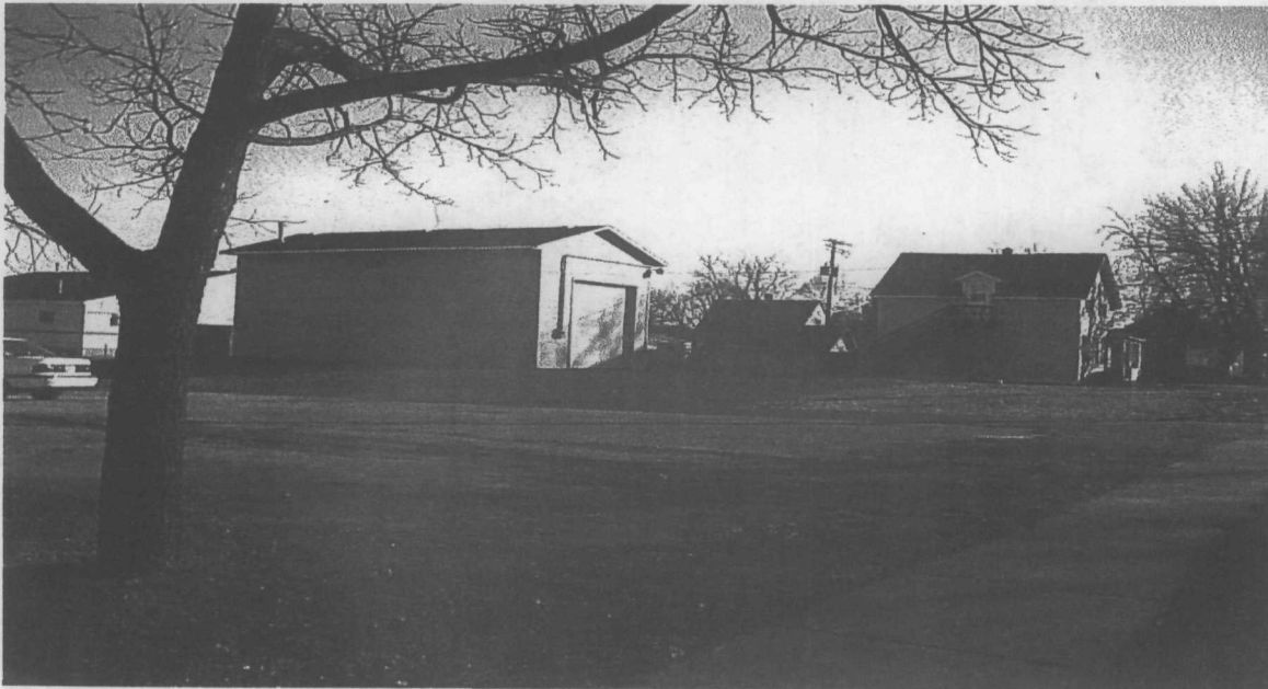
Relocated treatment building at Zinc Shop.
