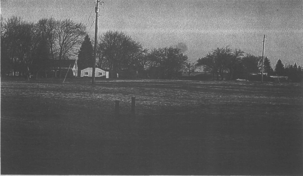
Final grade at Chrome Shop looking north from MW-107.
