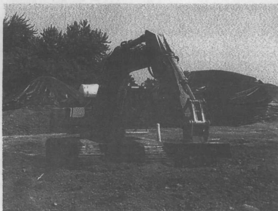
Backhoe with roto-tiller attachment
