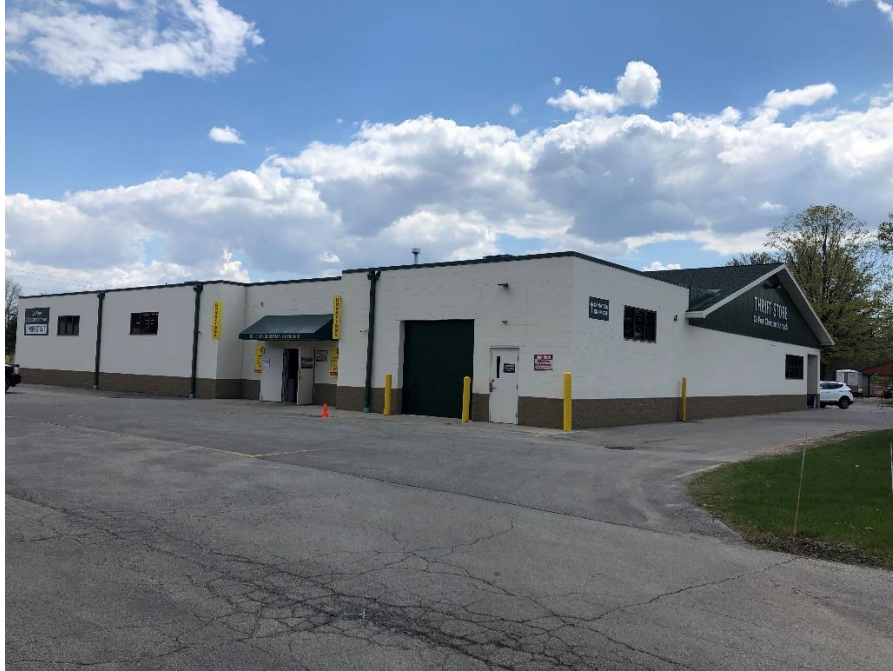
Photo 3 Description: building addition to resale shop Location: Zinc Shop
