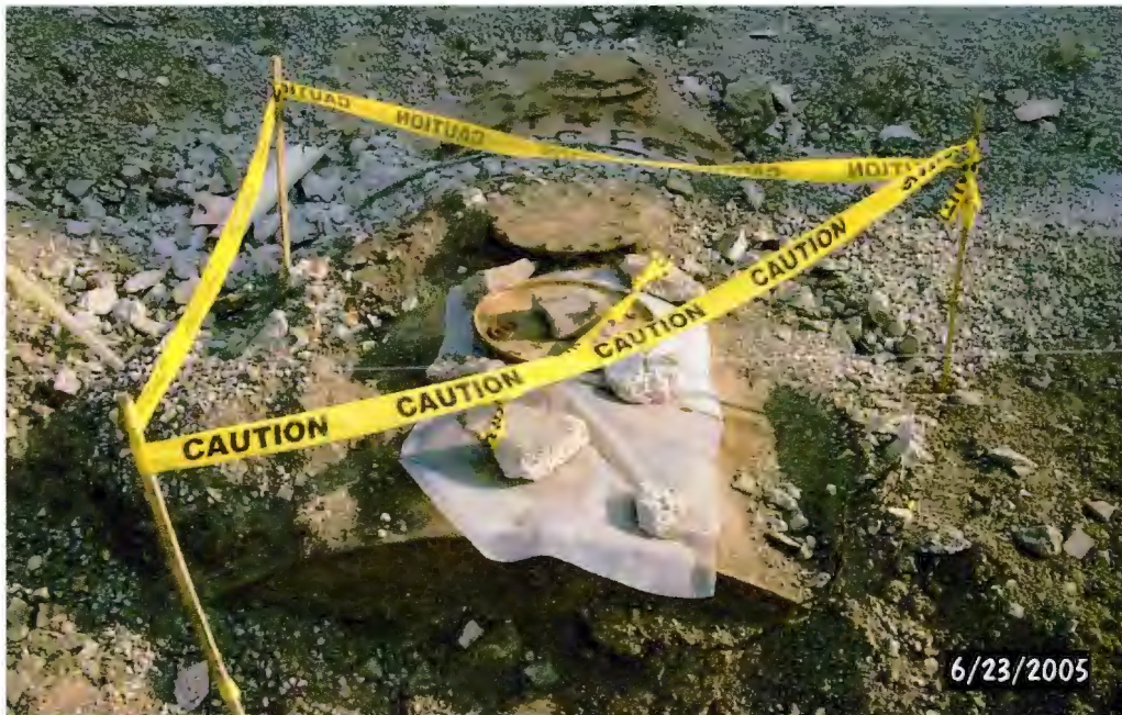
PHOTOGRAPH NO. 1: Uncovered UST– (facing north)
