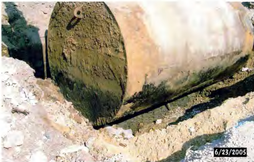
PHOTOGRAPH NO. 2: Excavated UST – (facing northwest)
