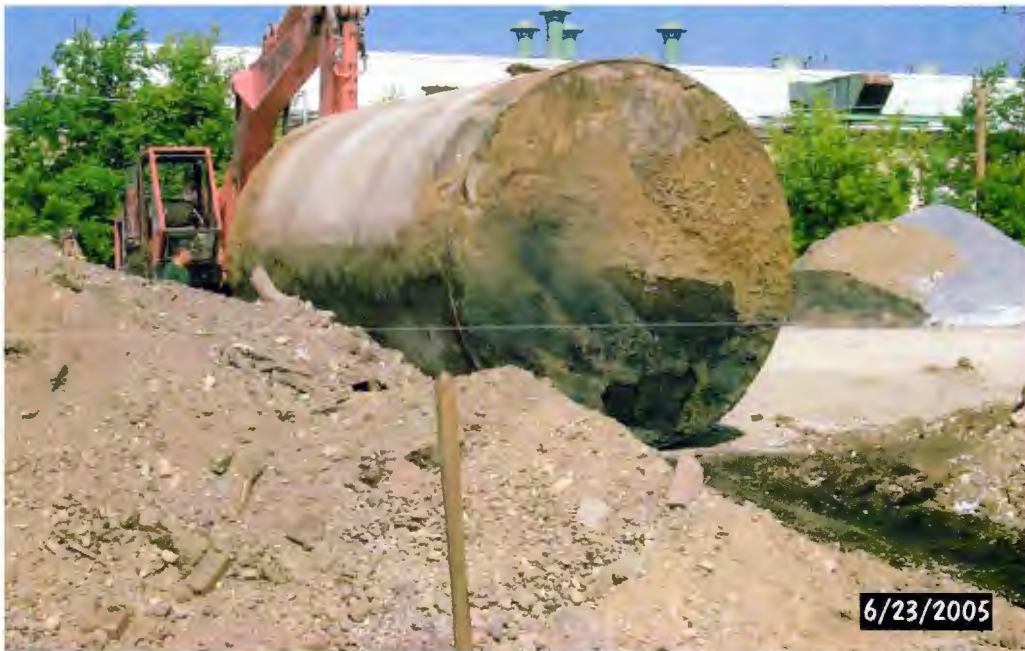
PHOTOGRAPH NO. 3: Excavated UST Removed From Cavity – (facing west)
