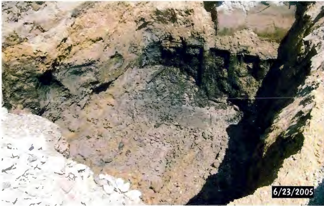
PHOTOGRAPH NO. 5: Extent of Soil Excavation – (facing northwest)
