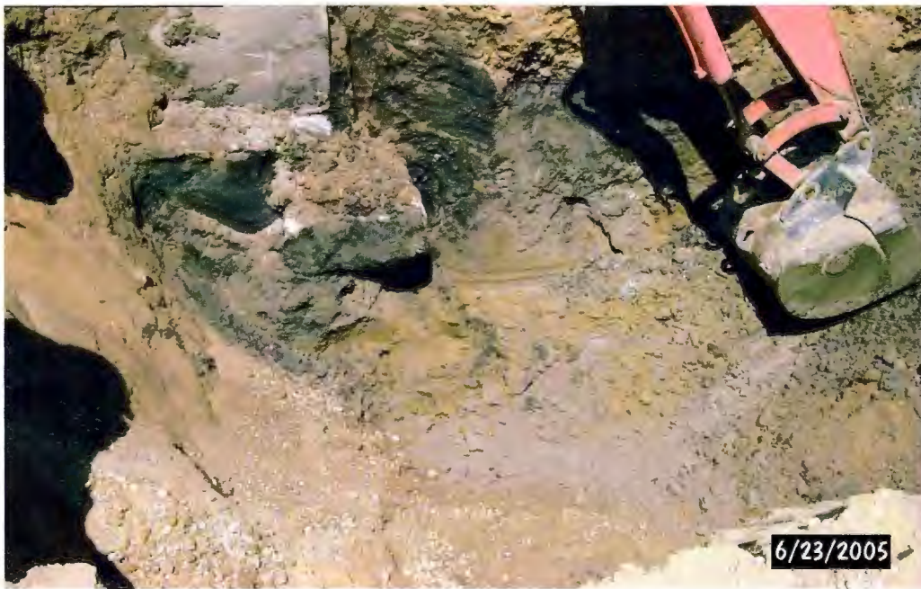
PHOTOGRAPH NO. 4: Soil Excavation Activities - (facing west)
