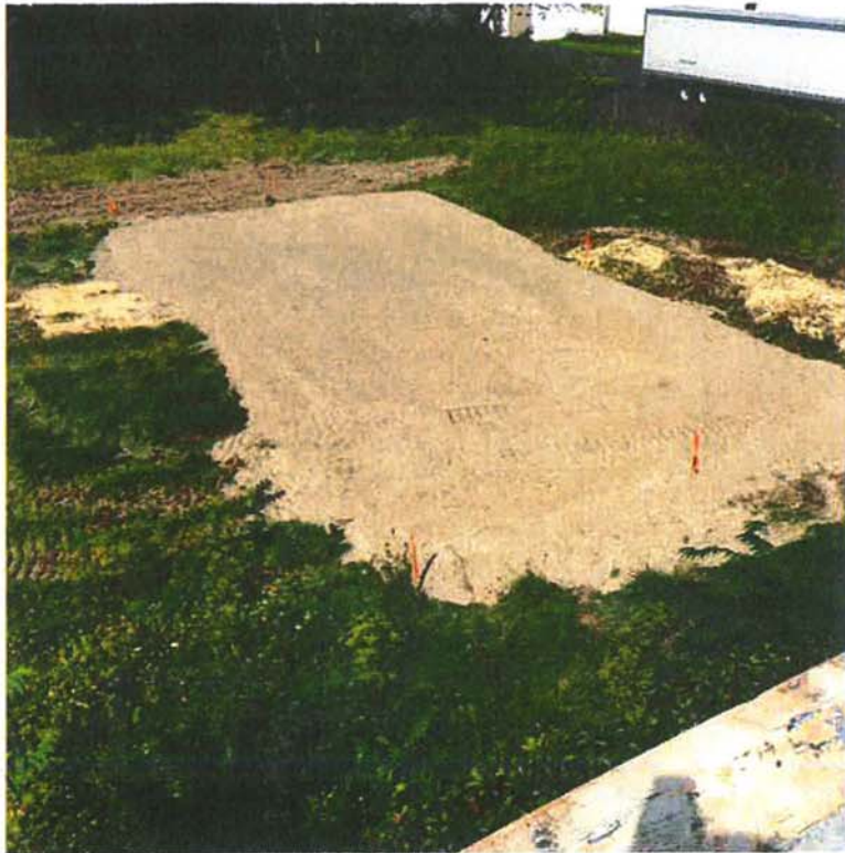
Figure 4 West view of the capped area.
