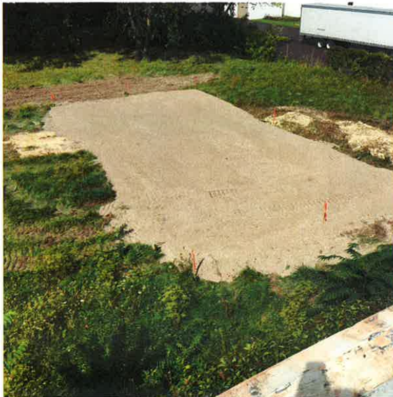
Figure 4 West view of the capped area.
