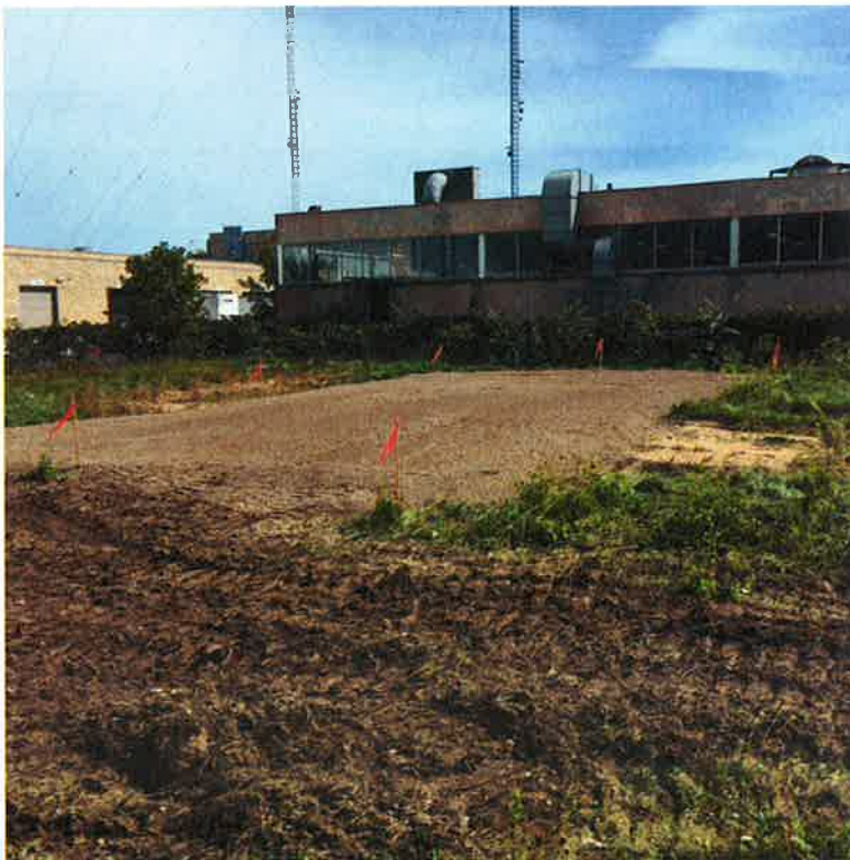
Figure 2 Northeast view of the capped area.
