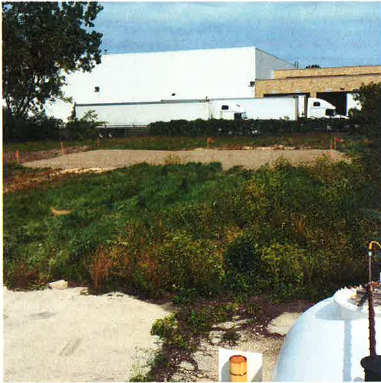
Figure 1 North view of the capped area.
