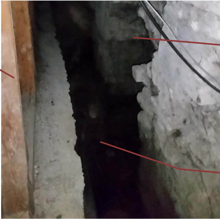
Photo 2. Gap (1.25 feet) between brick cribs and floor slab.
