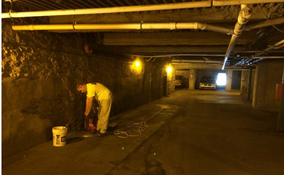
Photo 13. Coring through the slab at SS-3, looking east.
