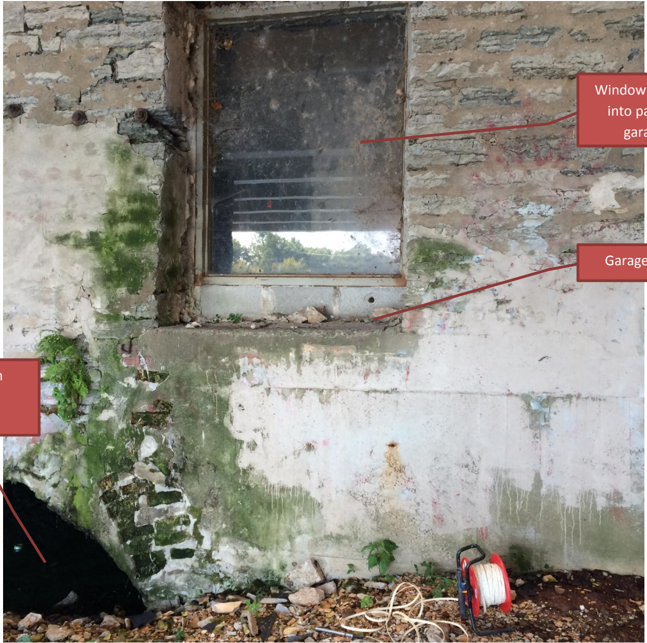
Photo 11. Looking west at the southeast corner of Building 415 from under Olde Oneida Street. The garage floor is approximately 4-feet above ground surface. There is no evidence of drainage structures however, archways like the one in the lower left of the photo extend west under the building and are filled with stagnant backwater from the Fox River Canal.
