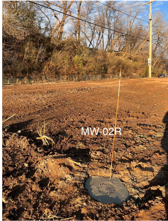
Photo 1: Well MW-02R converted to flush mount
