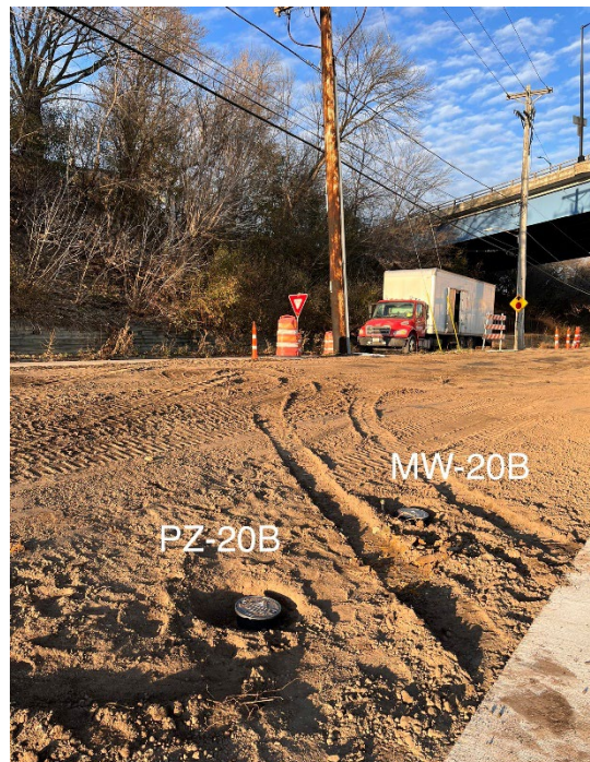
Photo 8: Wells PZ-20B and MW-20B converted to flush mount
