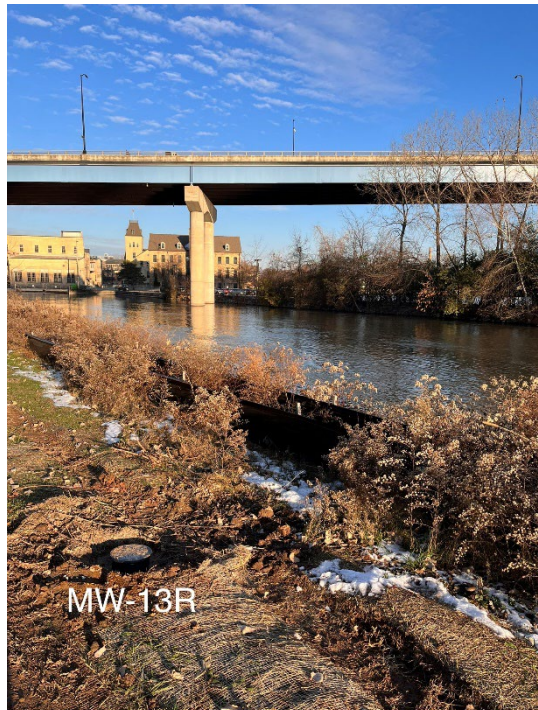
Photo 4: Well MW-13R converted to flush mount
