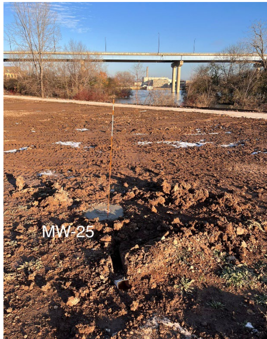
Photo 6: Well MW-25 converted to flush mount
