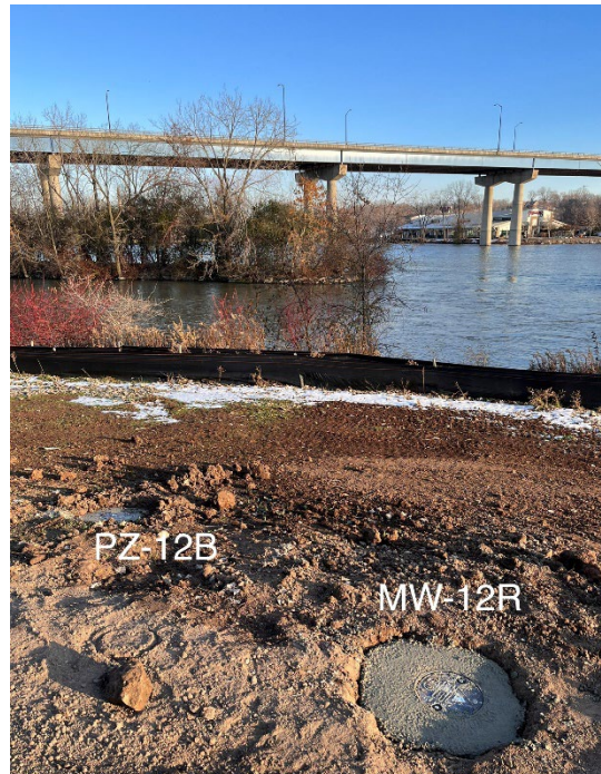
Photo 7: Wells PZ-12B and MW-12R converted to flush mount
