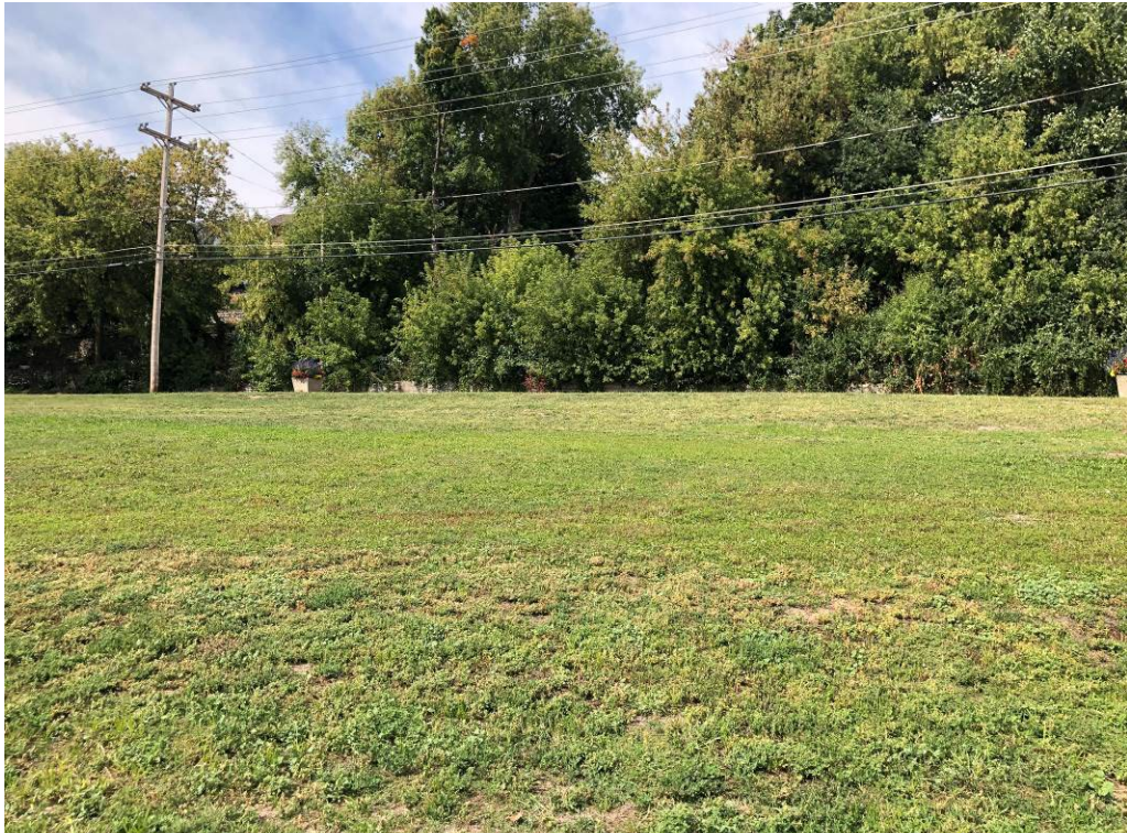
Photo 3: Central portion of Cap Maintenance Area looking north
