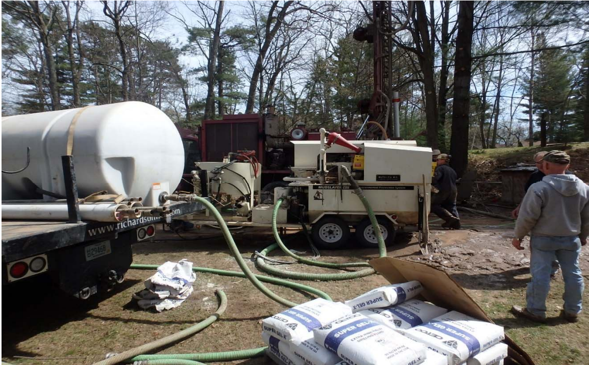
Photo 3 – Equipment for drill mud and borehole cuttings removal.
