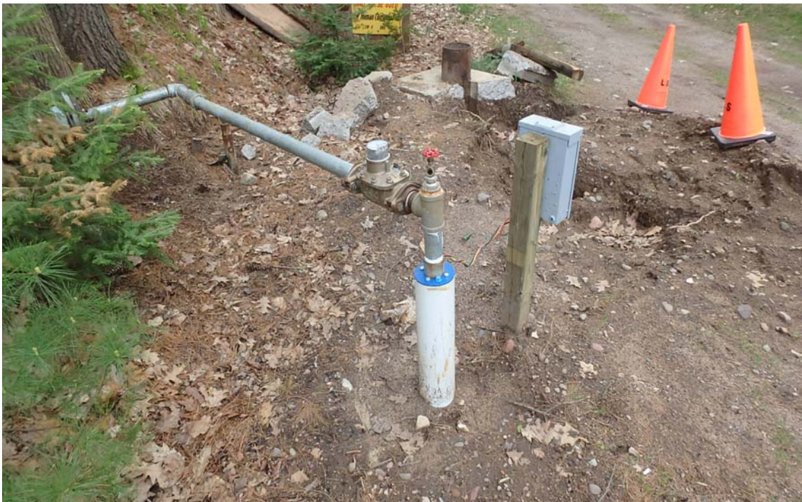
Photo 8 – New well EXW-4 on May 25, 2017 with old well in background and prior to surface restoration.
