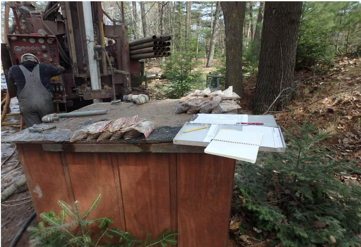
Photo 4 – Drill cuttings sampled every 5 ft during replacement well drilling on May 7, 2017.
