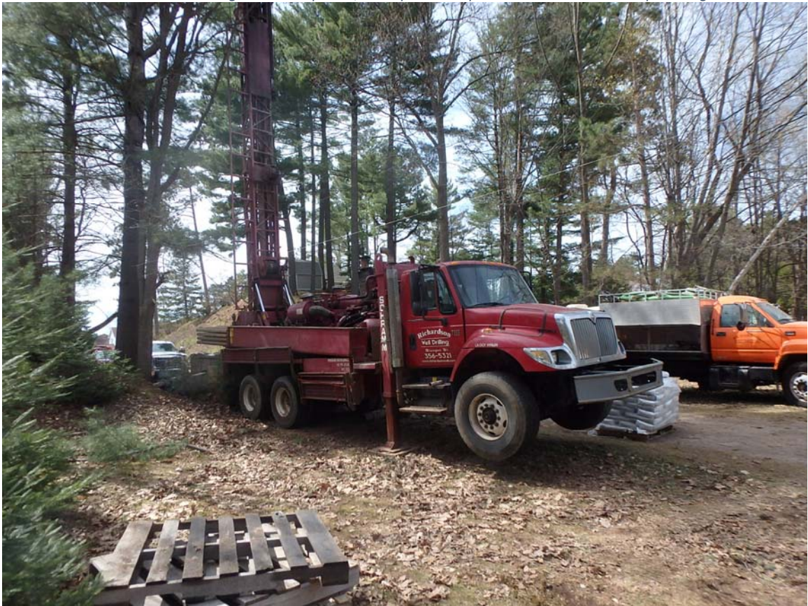
Photo 2 – Richardson Drilling installing new EXW-4 on May 7, 2017.
