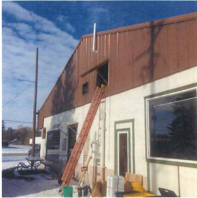
Photo 15: Attic access and discharge piping on main building.
