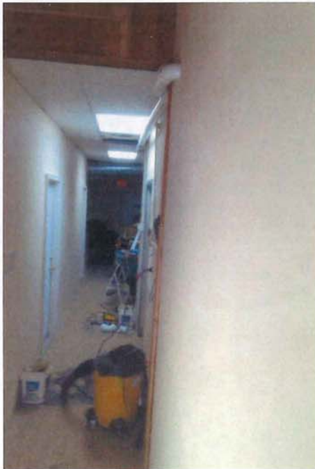
Photo 8: Piping connecting pickup points #2 and #3 in main building.
