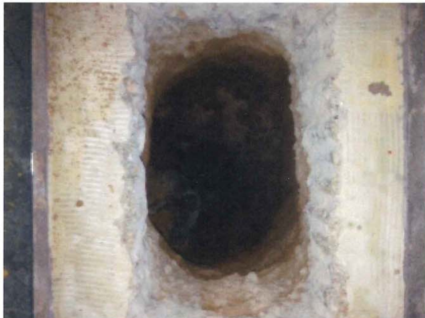
Photo 2: Pickup point #2 in storage unit 1 of main building – boulders at bottom.
