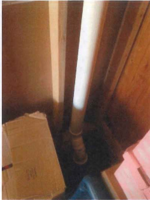
Photo 3: Pickup point #2 in storage unit 1 of main building – boulders at bottom.
