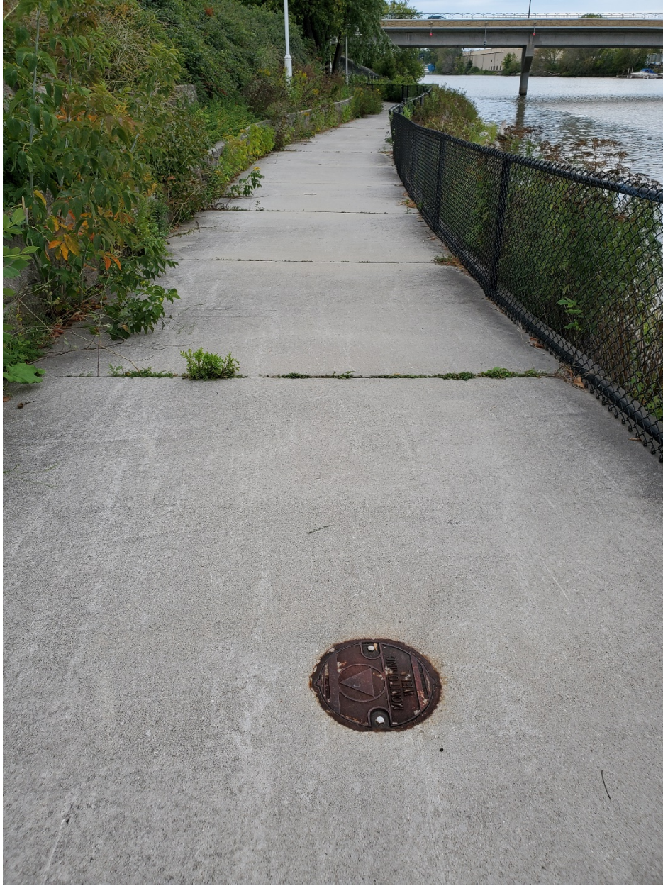
Photo 9: Possibly air sparge Well BW-08. Photo looking southeast from southeast end of site, taken September 21, 2022.
