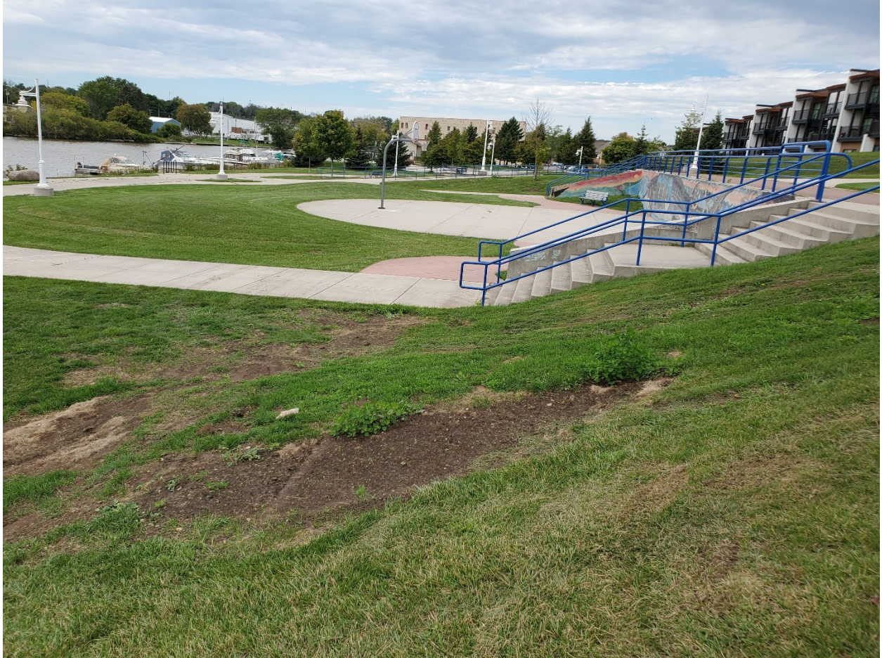
Photo 2: Re-seeded exposed soil on the top of the cover south of the basketball court looking northwest. New condominiums are in the upper right of photo. Photo taken September 21, 2022.
