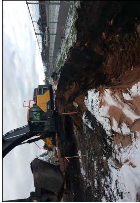
Excavating on north property line near B1
