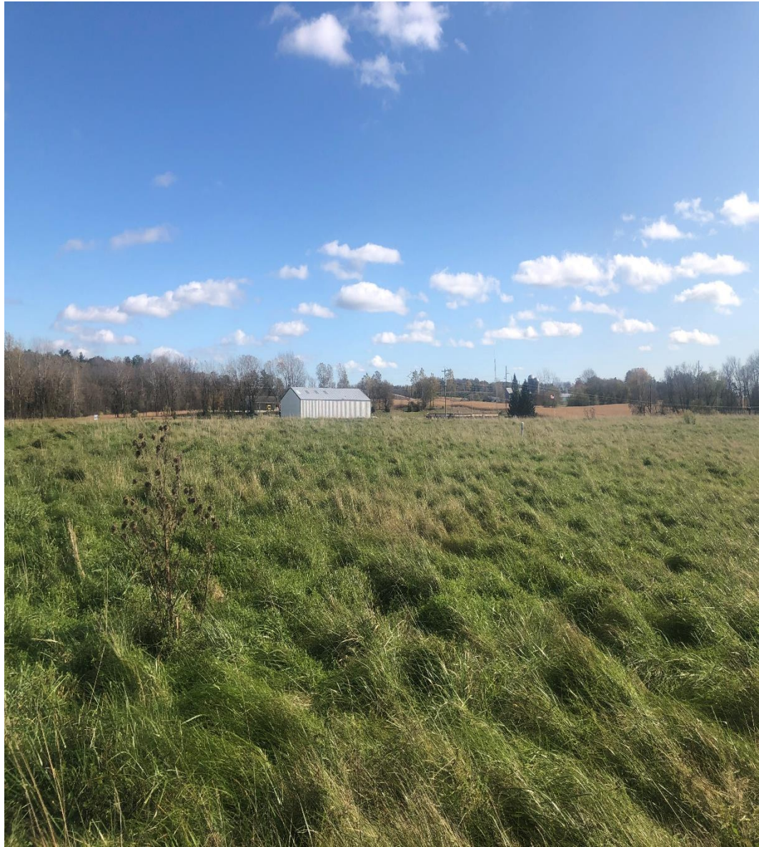
Photo showing remediation building where the out-of-service groundwater treatment machinery is housed and where the leachate from the LL was stored.
