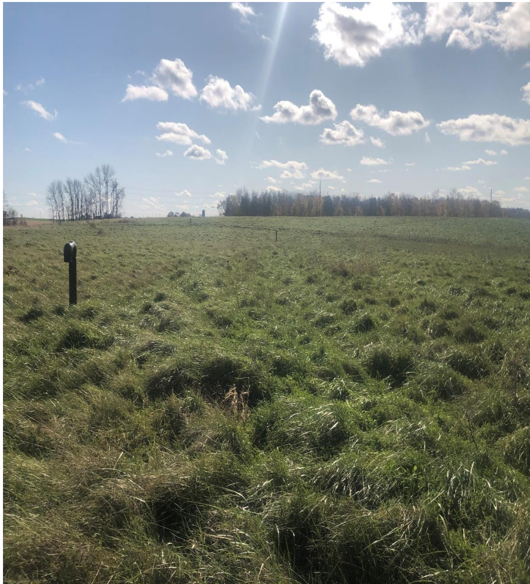
Photo from top of LTR landfill showing thick cover that is well maintained and mowed properly.
