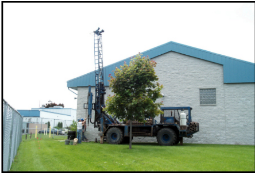
Photo 3 - Piezometer Installation at PZ5
