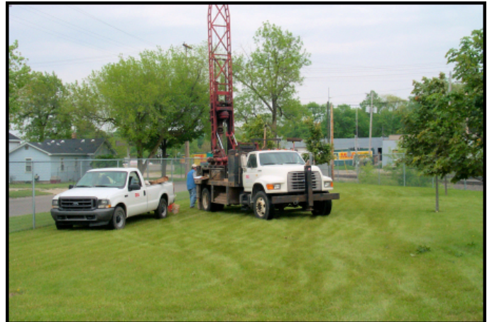
Photo 4 - Monitoring Well Installation at MW-111
