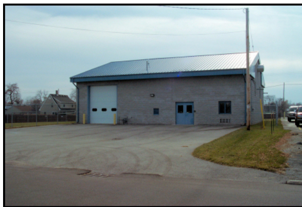
Photo 1 - Mauthe Treatment Facility
