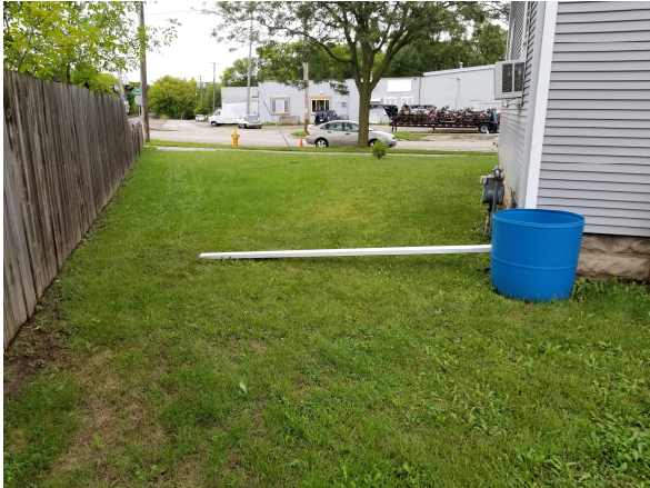
Photo #1 Looking east at the northwest roof drain.
