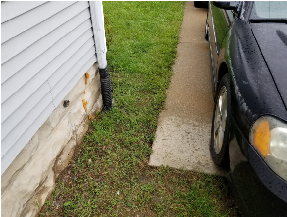
Photo #3 Looking east at the southeast roof drain.
