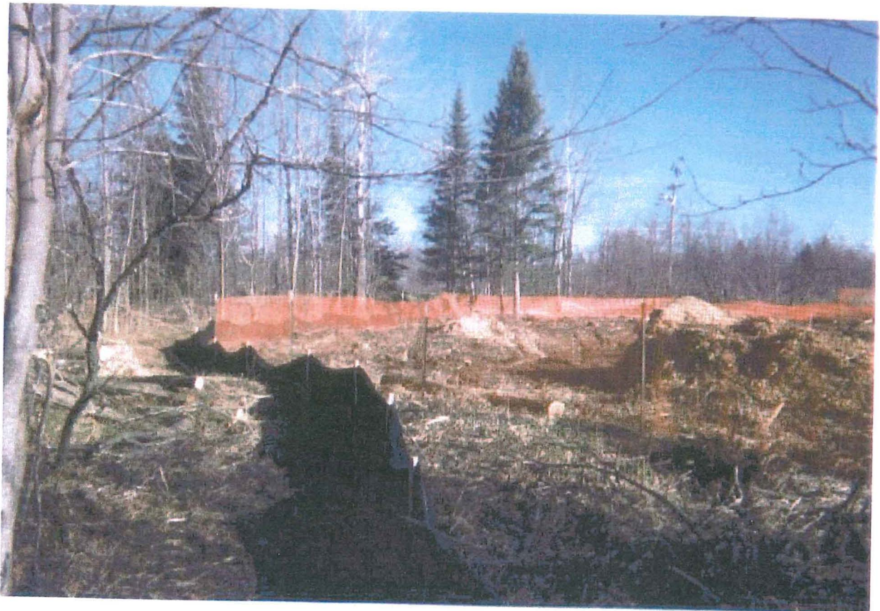
Photo 2: Installation of silt fence and safety fence prior to soil excavation.
