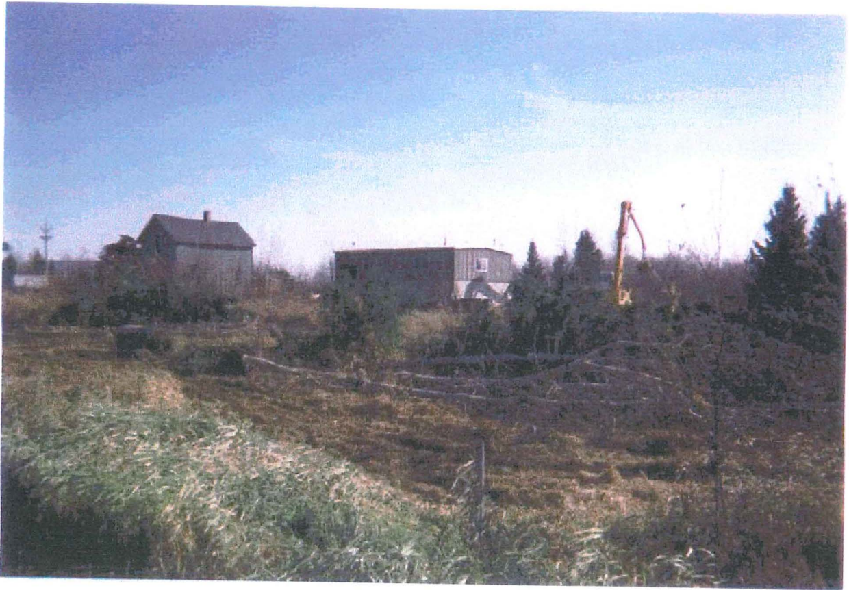
Photo 1: Clearing and grubbing activities prior to the start of construction.
