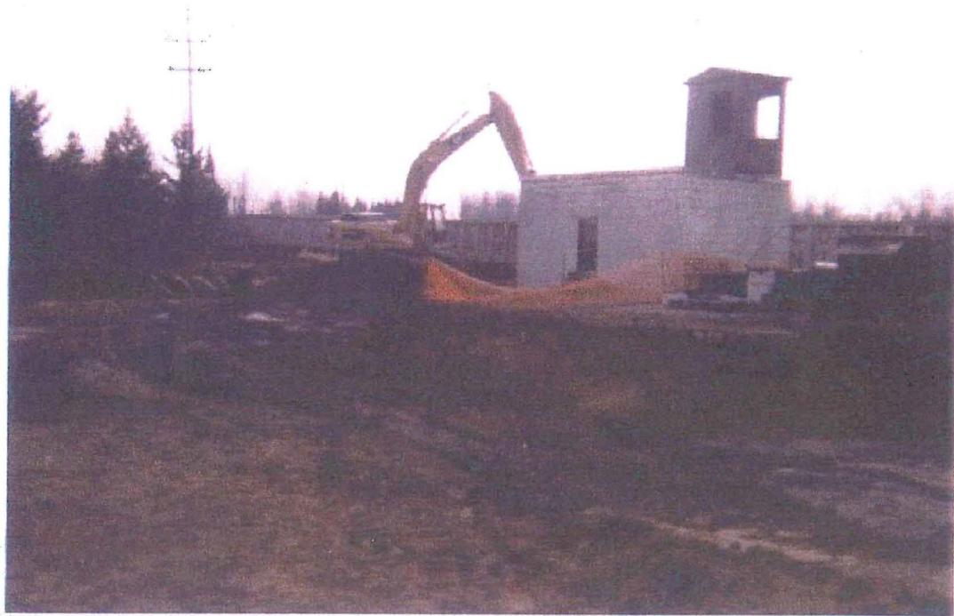
Photo 3: Excavation of soil above the site cleanup objective of 500 mg/kg.
