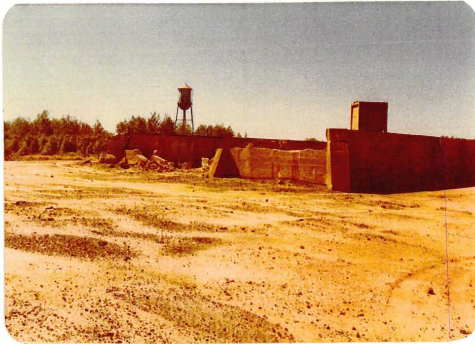
Sulfur Storage Bunker
