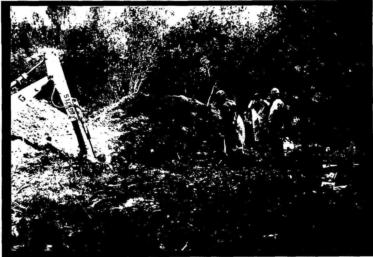
Photo 5: Closure Area 2 - During Excavation - August 25, 1998
