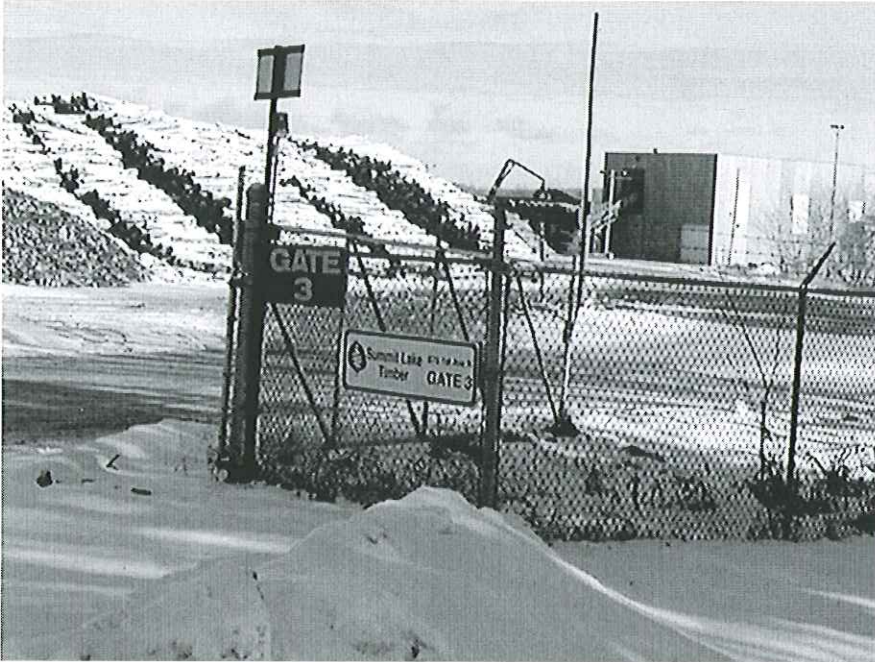
Flambeau Paper Mill Wood Yard (BRRTS # 02-51-000163) – Southwest corner of the site looking east. Note: fence and gate restricting site access. Site remains industrial use. 1/24/2007
