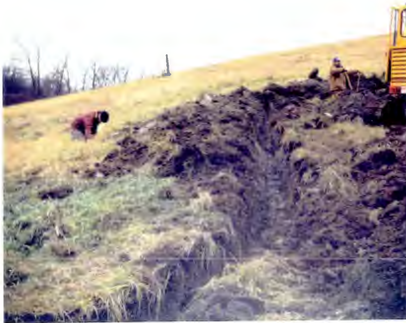
A View of the Trench for Electrical Conduits
