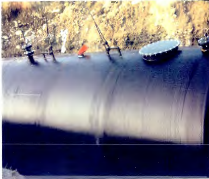
Placing the Tank in the Excavation
