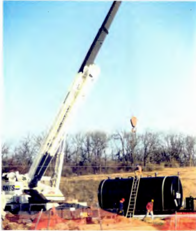
Unloading the Tank From the Trailer
