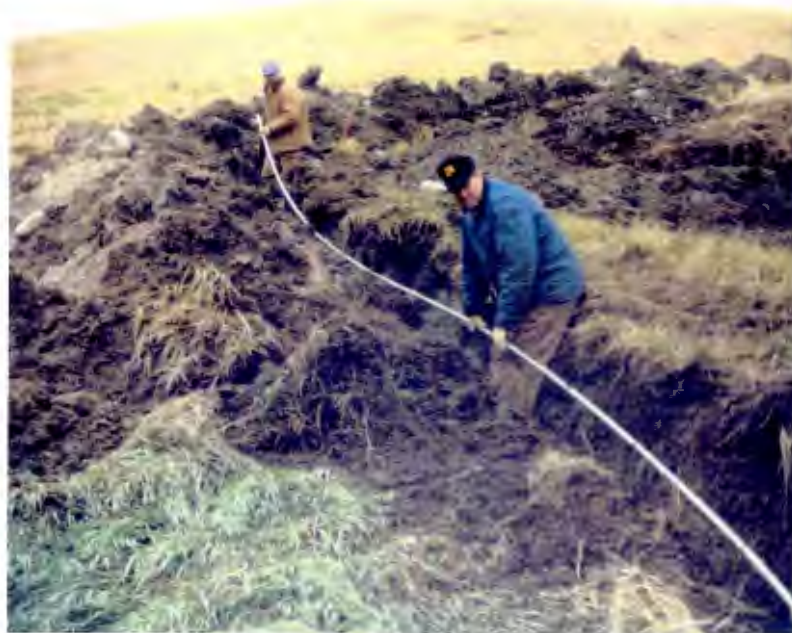
Laying the Conduit in the Trench
