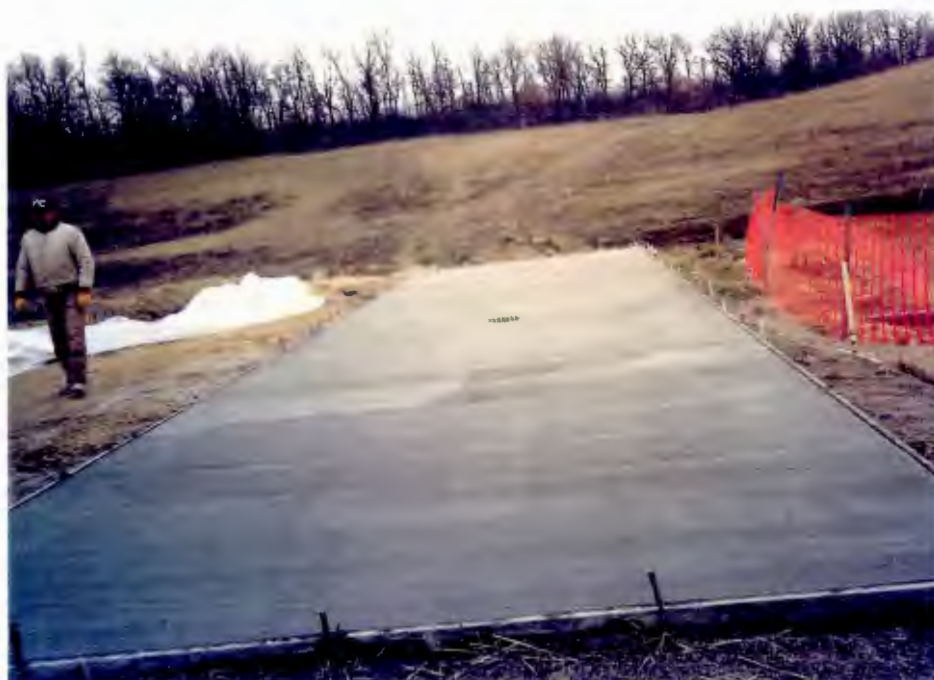
View of the Finished Concrete Slab
