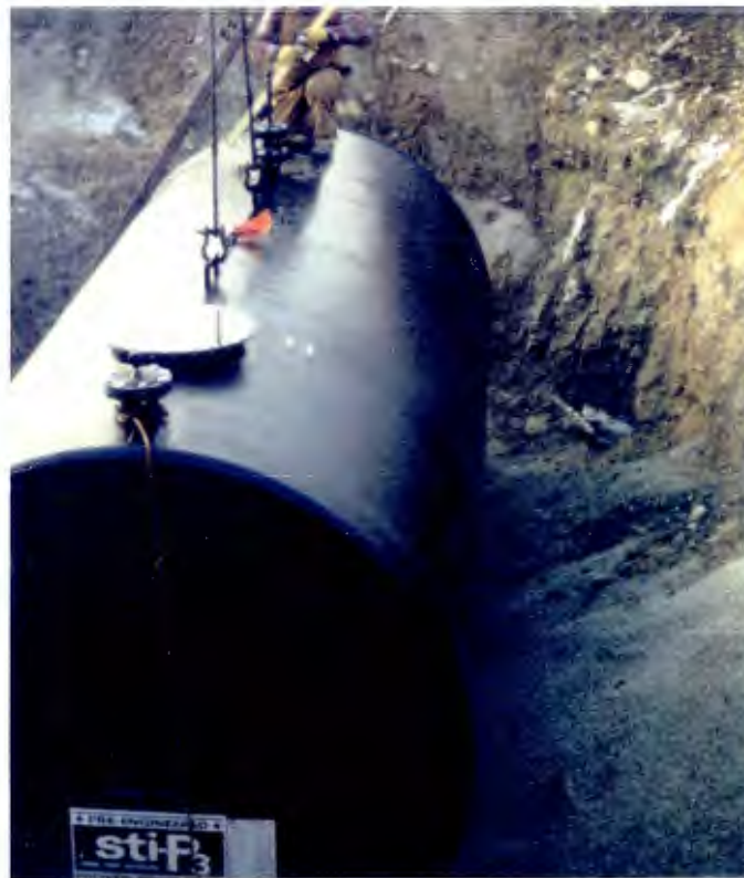
Checking the Level of the Tank, Prior to Anchoring
