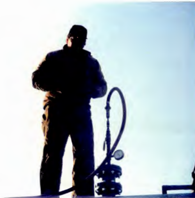
Air Testing of the Tank in Progress
