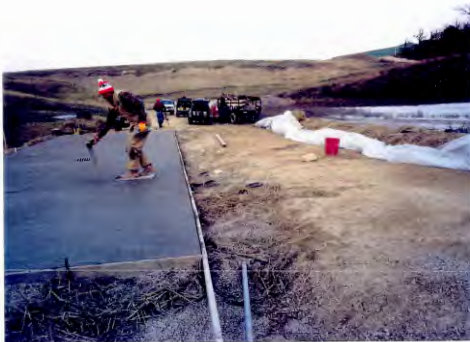
Construction of the Concrete Slab
