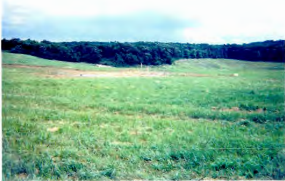
Photograph 1: Area Staked Out for Backfilling
