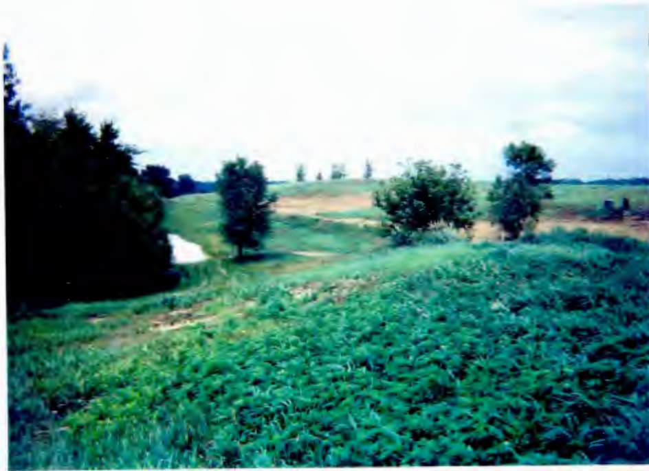
Photograph 4: Finished Western Edge Prior to Reseeding
