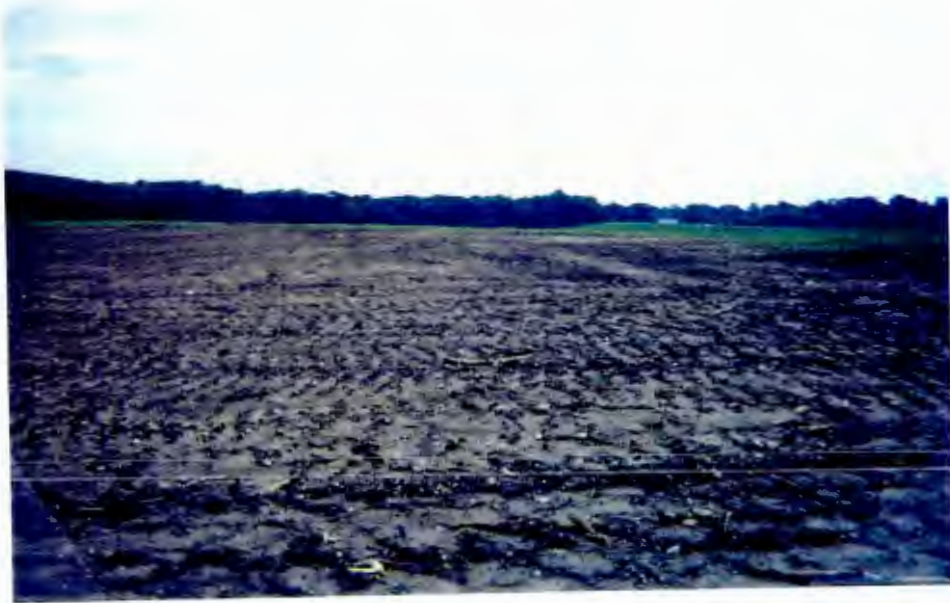
Photograph 3: Closeup of Compacted Fill Area
