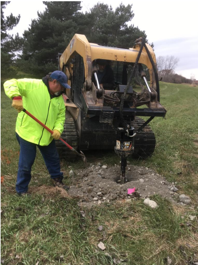
11/28/17 soil boring, stationing 2+50, looking east.
