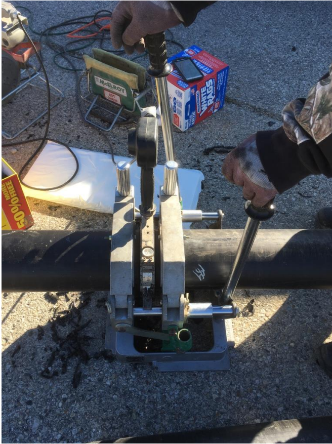
11/29/17 new 6 inch diameter by-pass header pipe, butt fusion welded.
