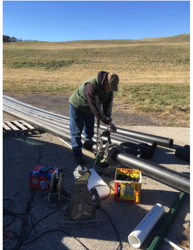
11/29/17 new 6 inch diameter by- pass header pipe, butt fusion welded.
