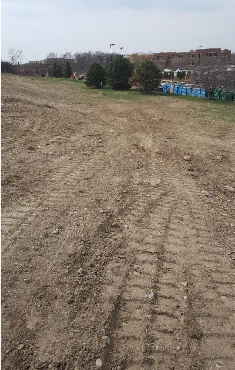
May 1, 2018 Grading of bypass trench near stationing 2+50, looking northwest.
