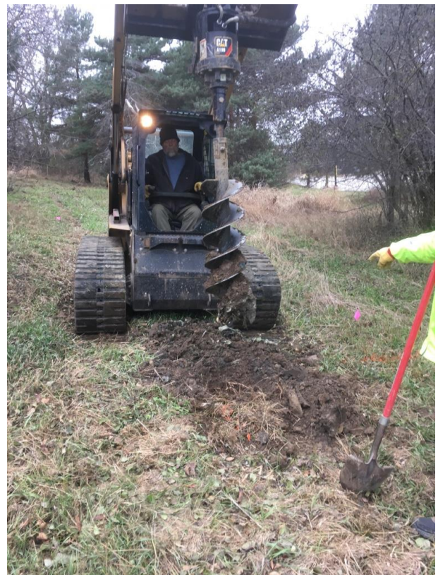
11/28/17 soil boring, stationing 5+00 looking west.
