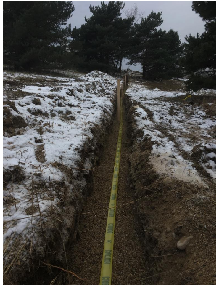
12/11/17 stationing 5+30, by-pass header pipe backfilled with pea gravel looking west.
