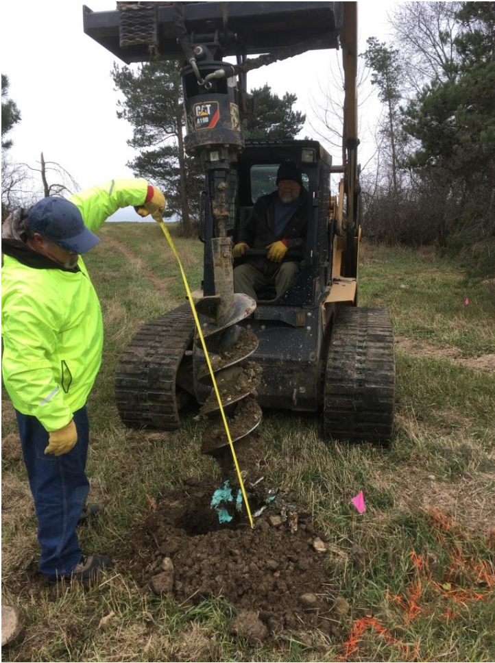
11/28/17 soil boring, stationing 5+00, looking south.
