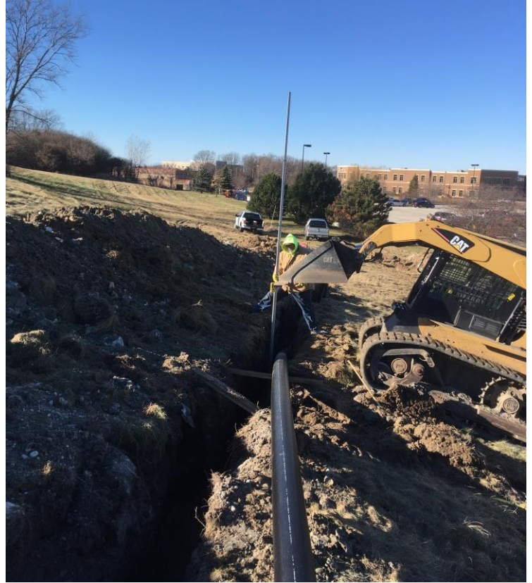
12/6/17 Near stationing 2+00 looking northwest. 6 inch by-pass pipe being placed in trench.
