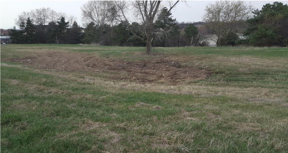
Settlement Area 1 – Looking North - After filling and regrading.
