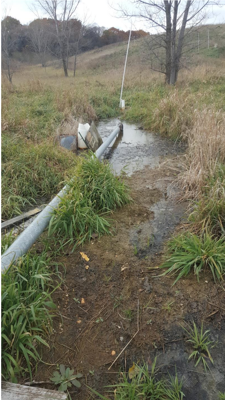
10,000 gallon UST leachate load out tank before drain tile installed (November 2018)
