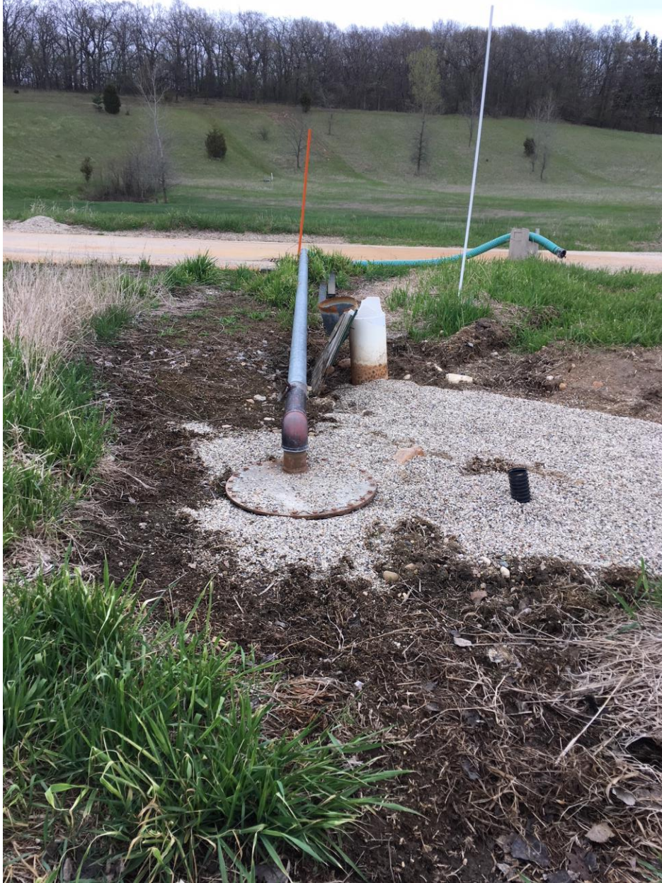
10,000 gallon UST leachate load out tank after drain tile installed (December 2018)
