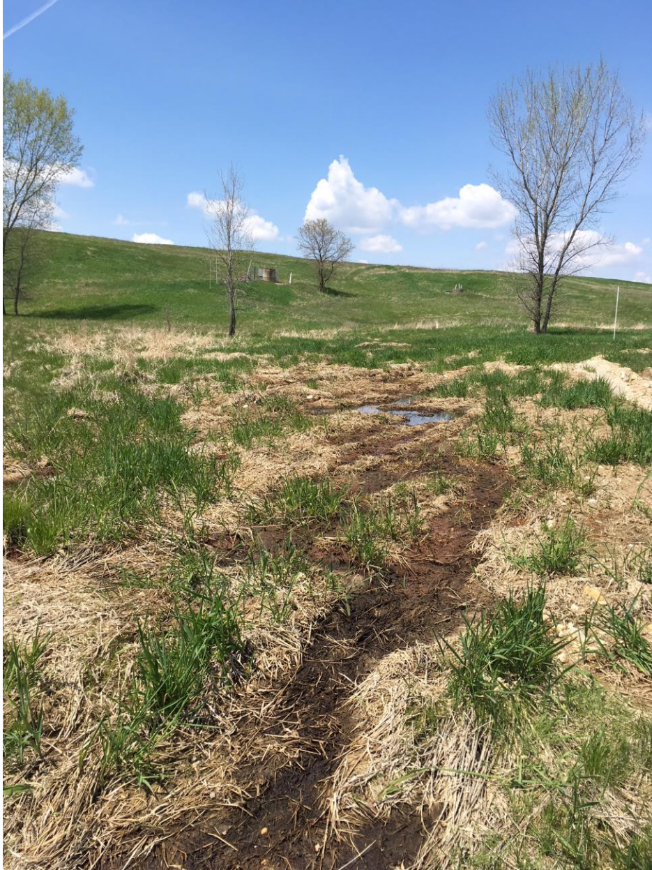
Leachate seep near leachate load-out area (May 2019)
