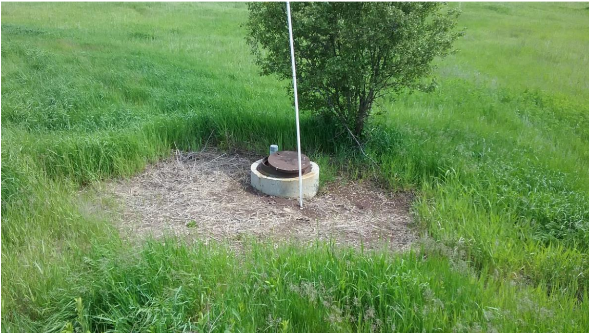
Photo #7: Gas Well G-3 - Stressed Vegetation Surrounding Gas Well
