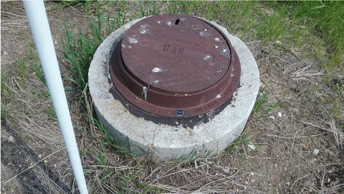
Photo #10: Gas Well G-8 Lid
