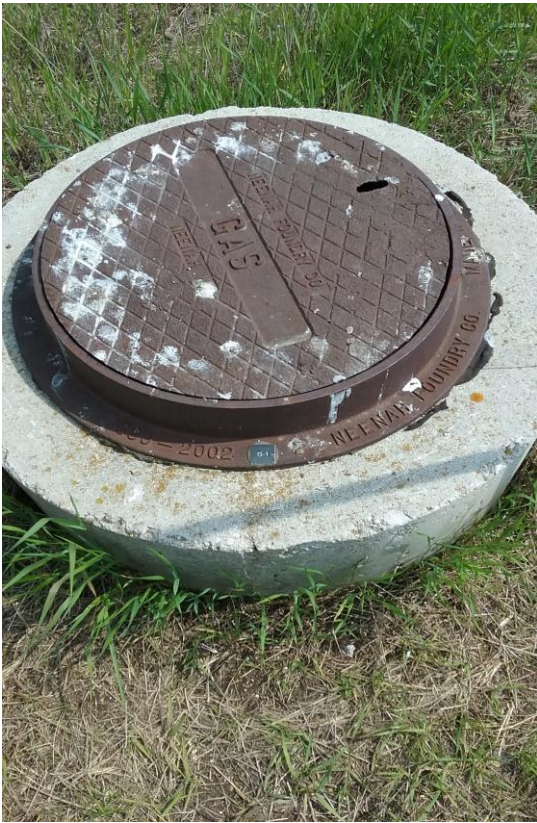
Photo #1: Gas Well G-1 Lid
