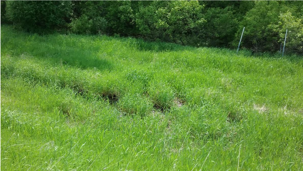
Photo #14: Picture Of Low Wet Area West Side Slope Near CS-02.
