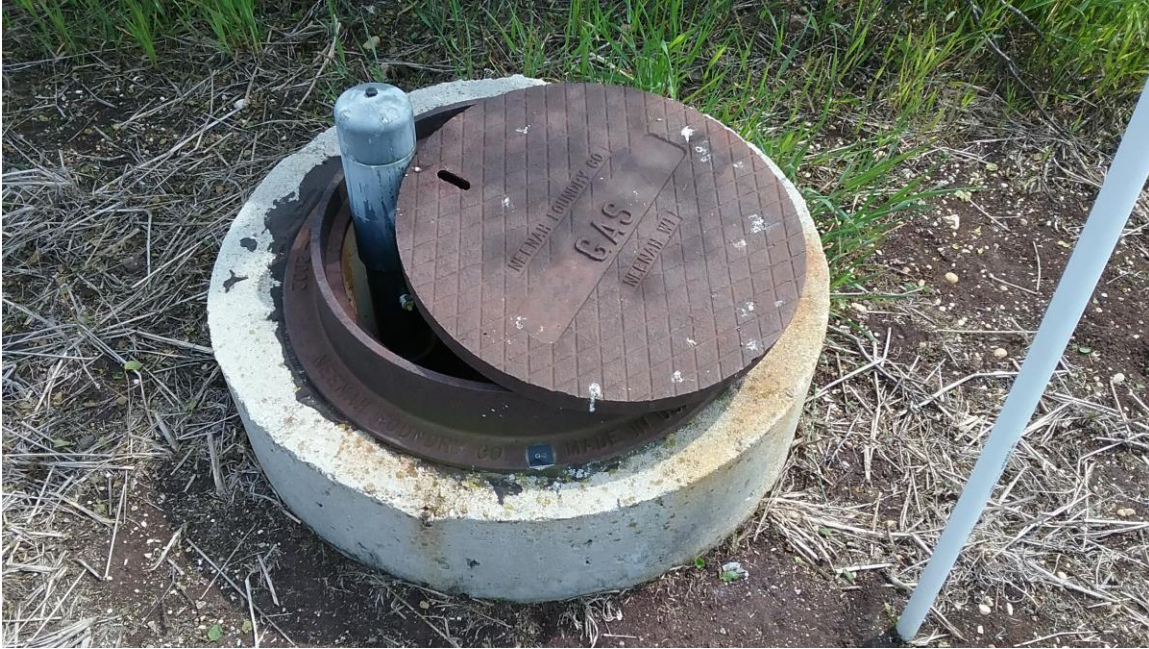
Photo #6: Gas Well G-3 Lid
