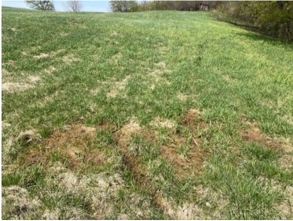
Photo #7 View vegetated cap condition (western portion of the landfill).
