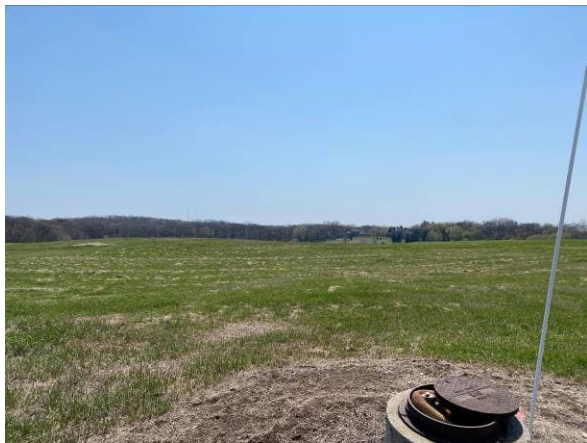
Photo #3 View of vegetated cap condition (south central portion of landfill)
