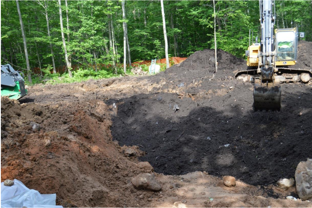
6/17/15: Beginning to backfill deep excavation, looking west
