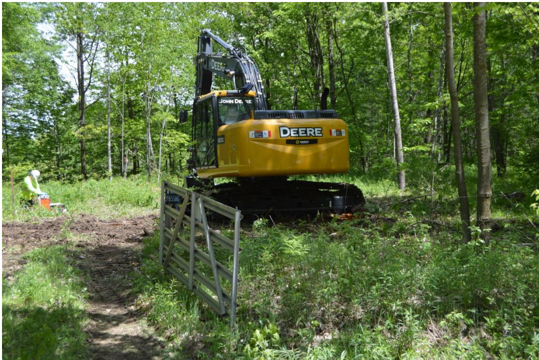
6/2/15: Preparation of site and backhoe for removal activities, looking north
