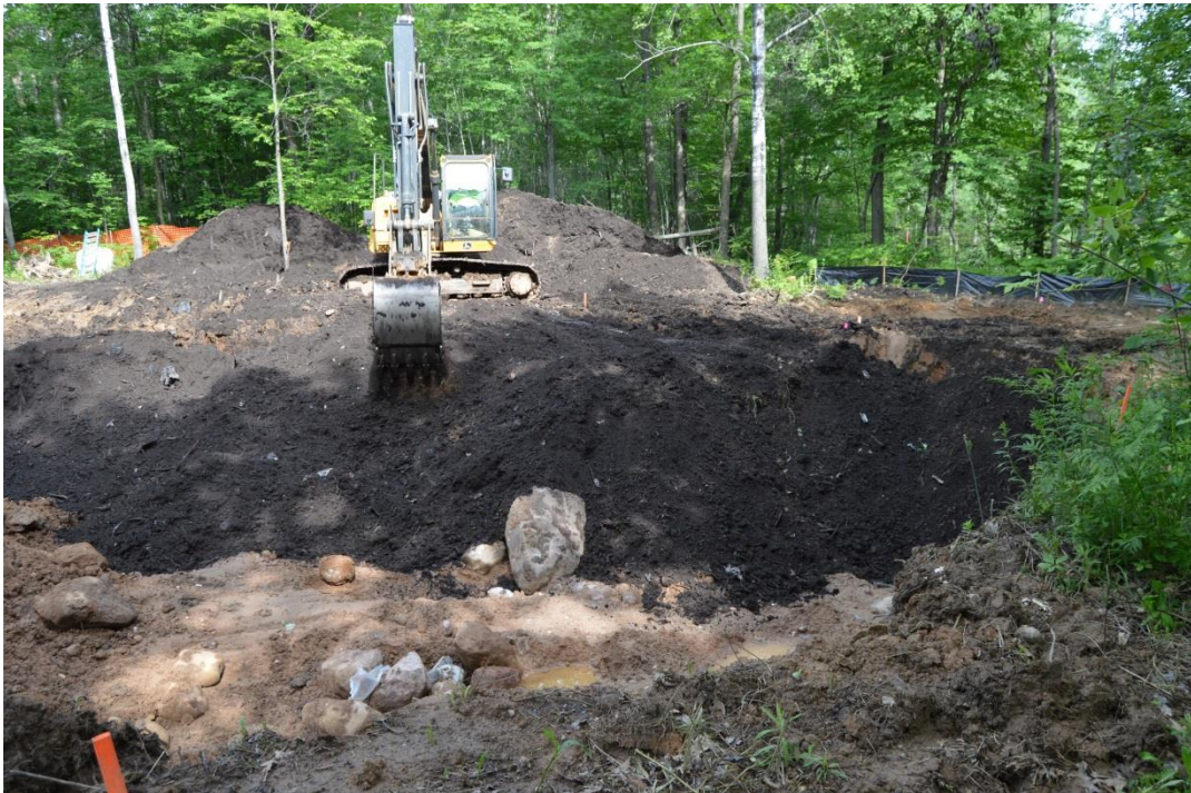
6/17/15: Beginning to backfill deep excavation, looking northwest
