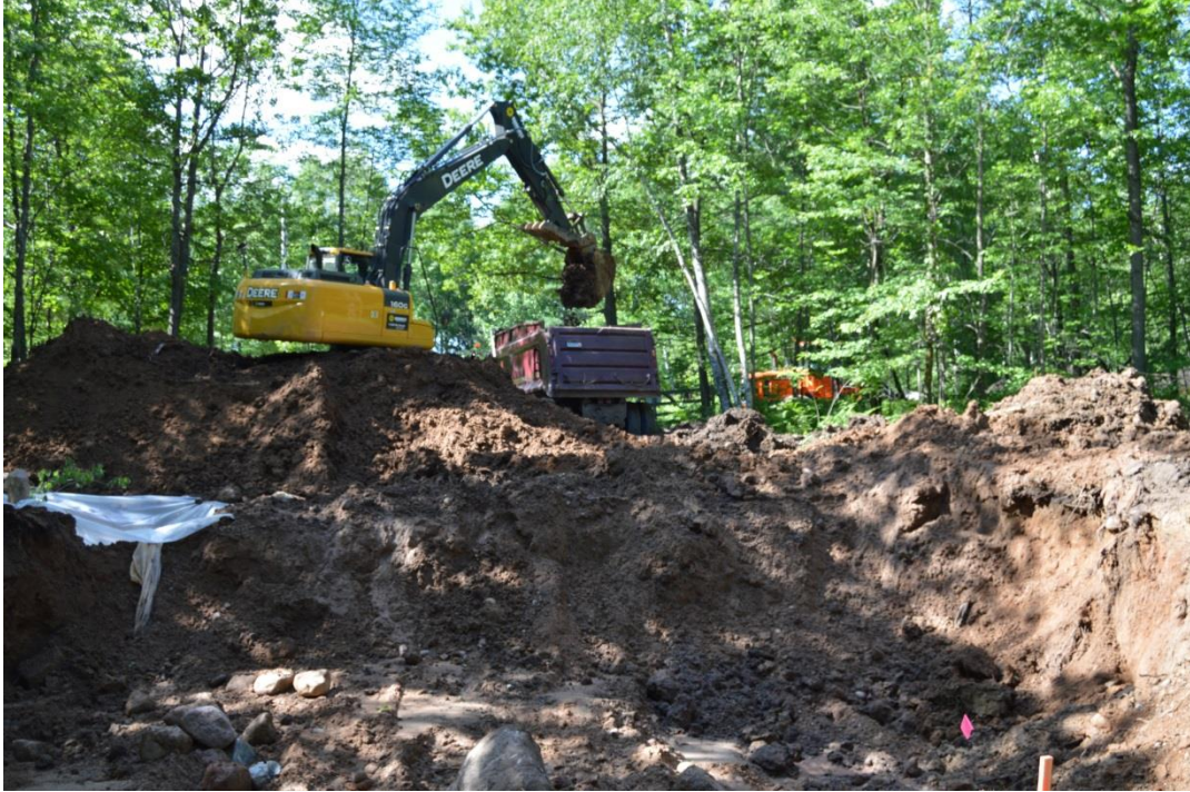
6/16/10: Loading out trucks with treated soil, looking south-southwest
