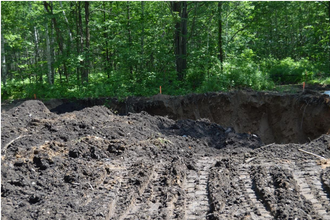
6/17/15: Beginning to backfill deep excavation, looking east
