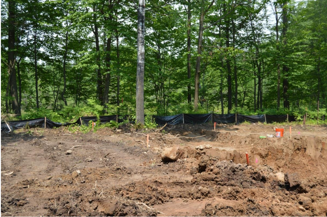
6/9/15: Silt fence with marsh in background, looking north
