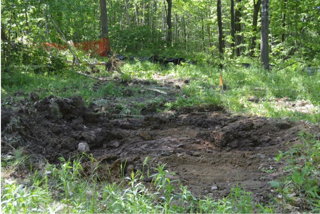
6/2/15: Begin excavating for collection soil sample for TCLP analysis, looking north-northwest
