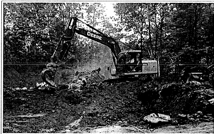
Contributed Photo Crews for the U.S Environmental Protection Agency are shown in the town of Aniwa last month excavating and removing more than 1,000 tons of contaminated soil from an old arsenic depot site.
