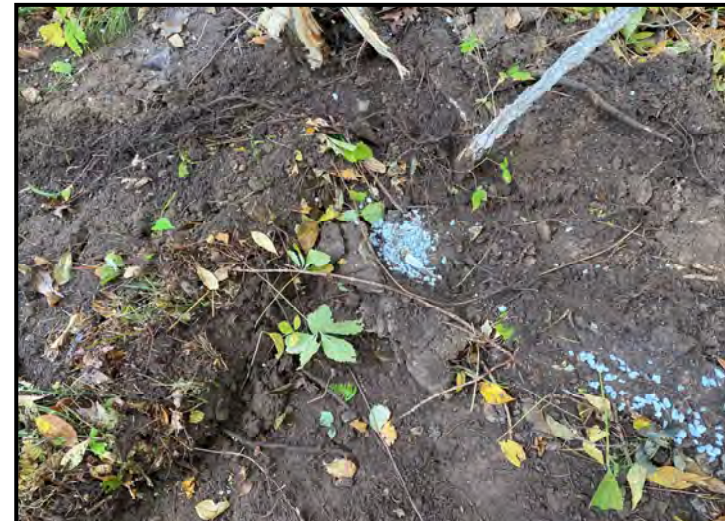
Abandoning monitoring wells
