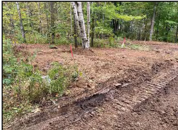
Clay cap placed and compacted
