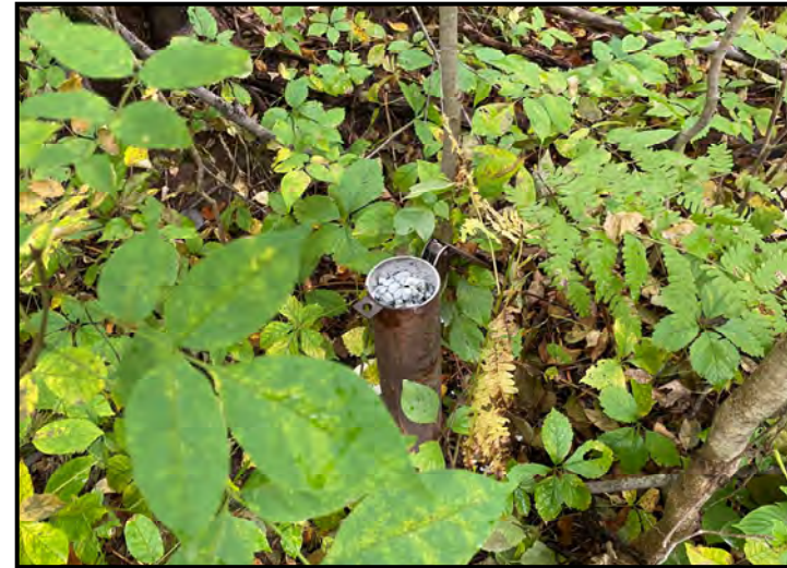
Abandoning monitoring wells
