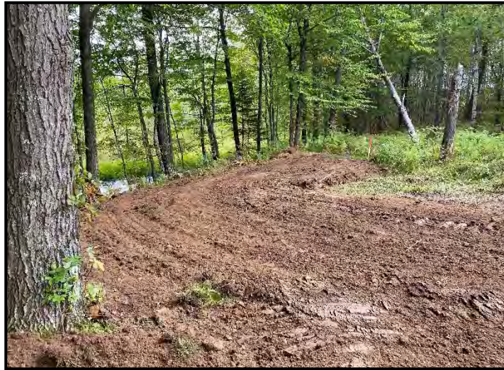
Clay cap placed and compacted
