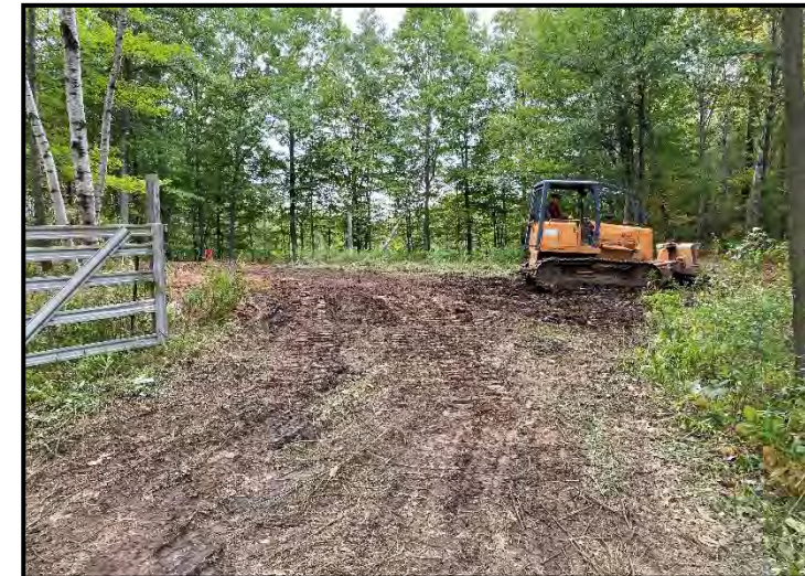
Capping prior to seeding
