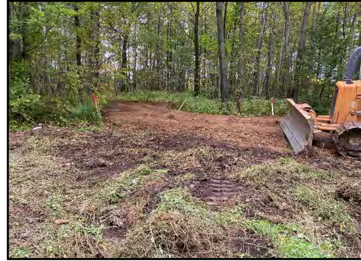
Clay cap placed and compacted
