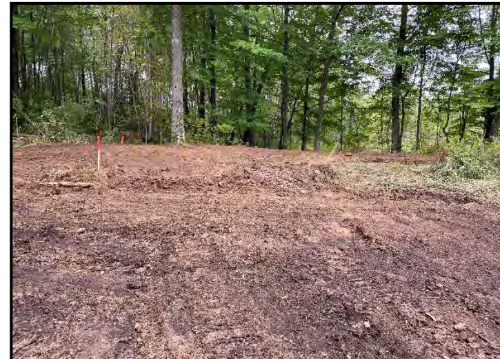
Clay cap placed and compacted
