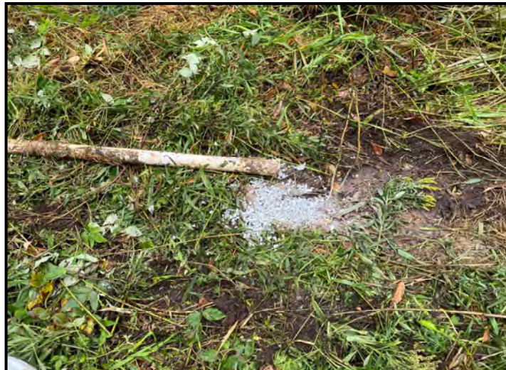
Abandoning monitoring wells
