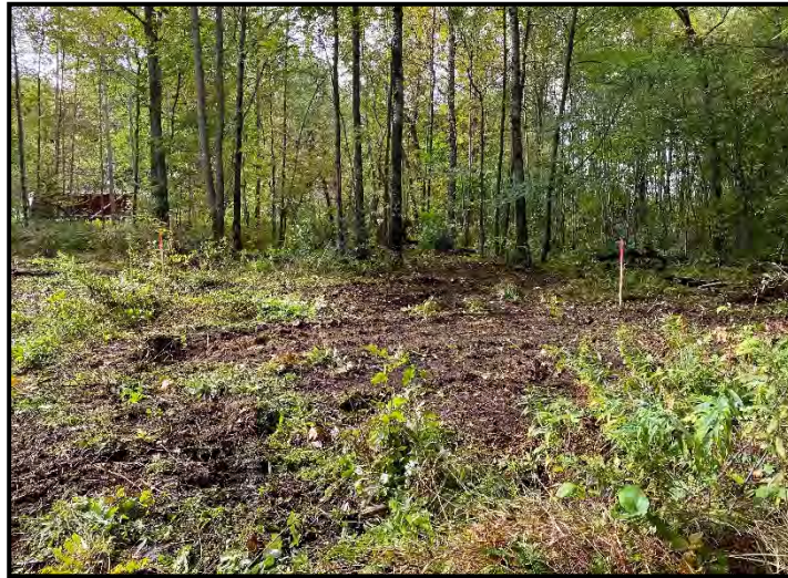
Stripping surface cover prior to capping
