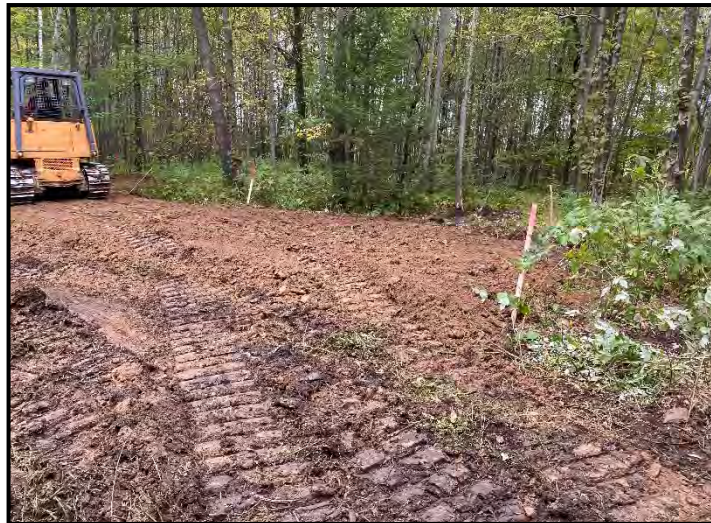
Clay cap placed and compacted
