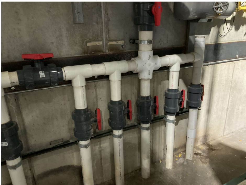
Title: Desmond's Men's Wear/0232000203/20220926/right bank of VMS manifold piping - all valves open
