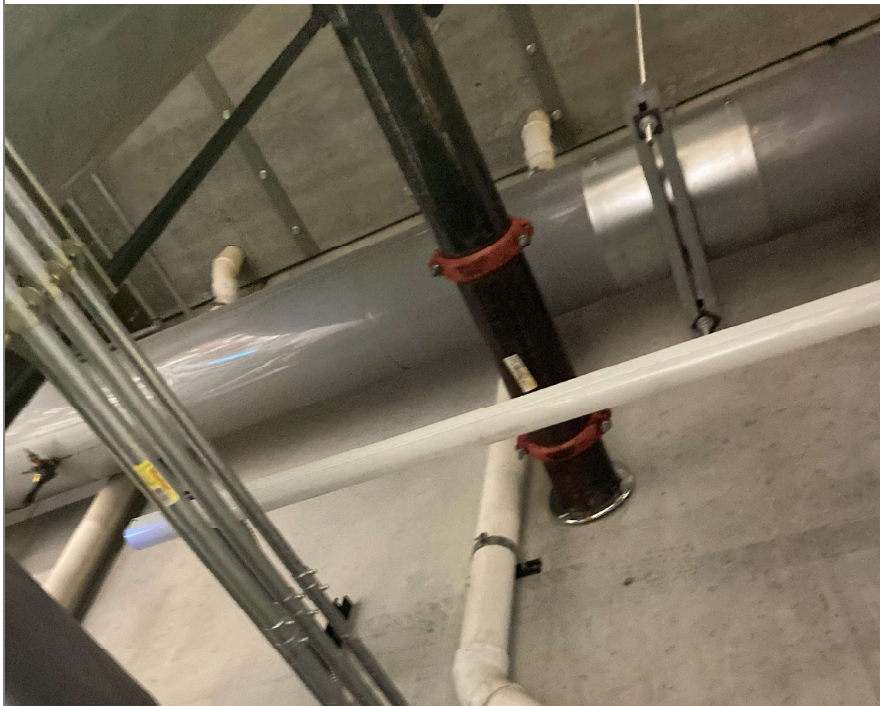
Title: Kwik Trip Bakery Expansion/0632560495/20220926/VMS piping to roof
