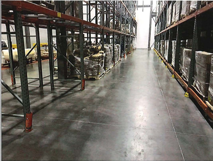
Title: concrete floor in good condition
