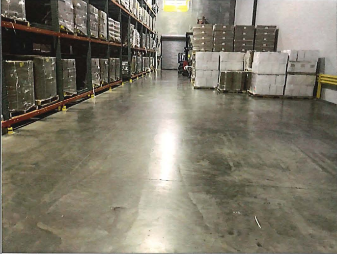
Title: Concrete floor in good condition
