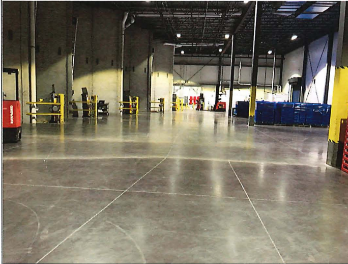
Title: Concrete floor in good condition
