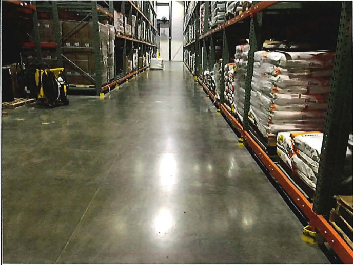
Title: Concrete floor in good condition
