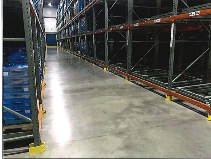
Title: Concrete floor in good condition
