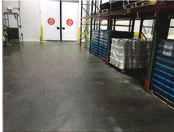
Title: Concrete floor in good condition
