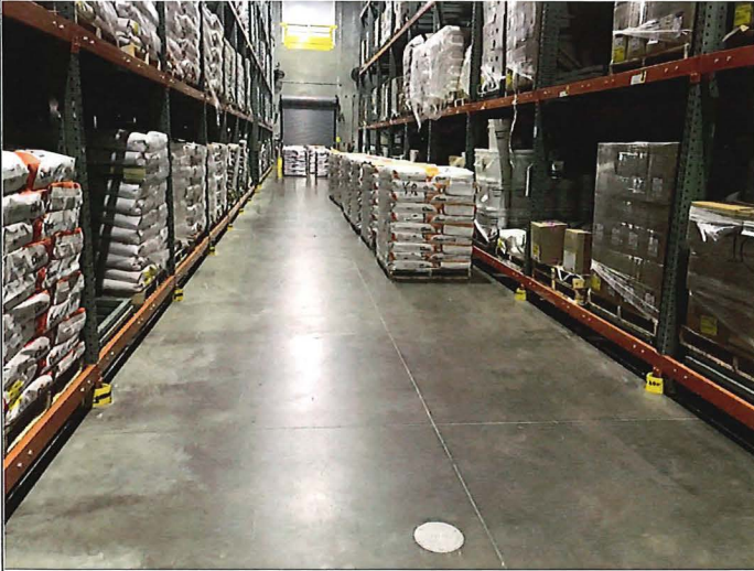
Title: Concrete floor in good condition
