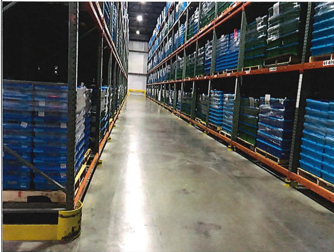
Title: Concrete floor in good condition
