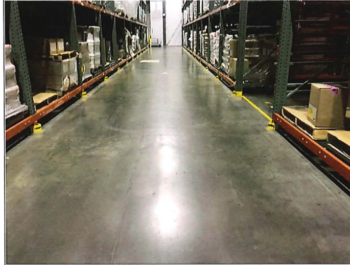
Title: Concrete floor in good condition
