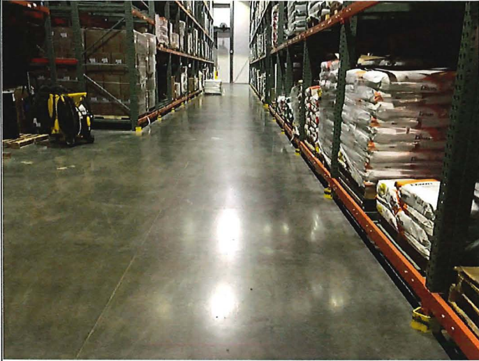
Title: Concrete floor in good condition
