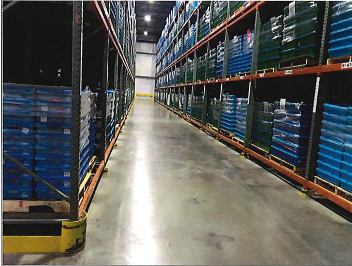
Title: Concrete floor in good condition
