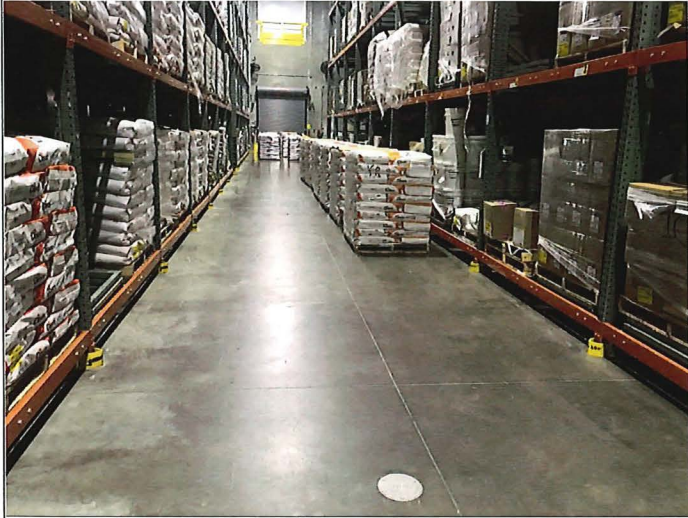
Title: Concrete floor in good condition
