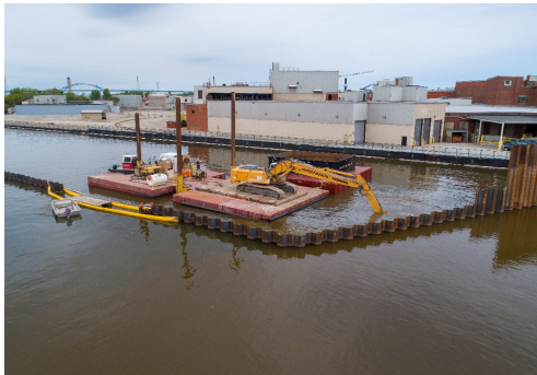
Mechanical Dredging Operations
