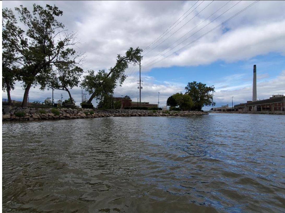
Upstream extent, Western shore.
