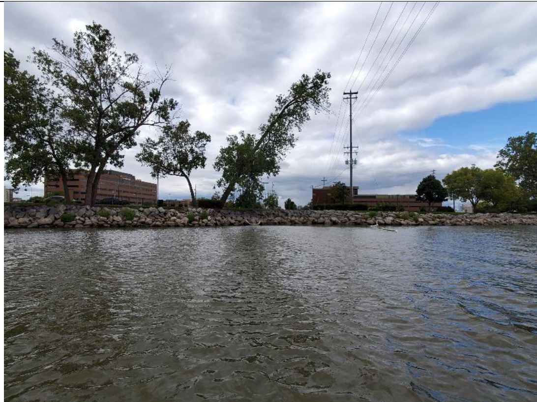
Across waterway view of western shoreline
