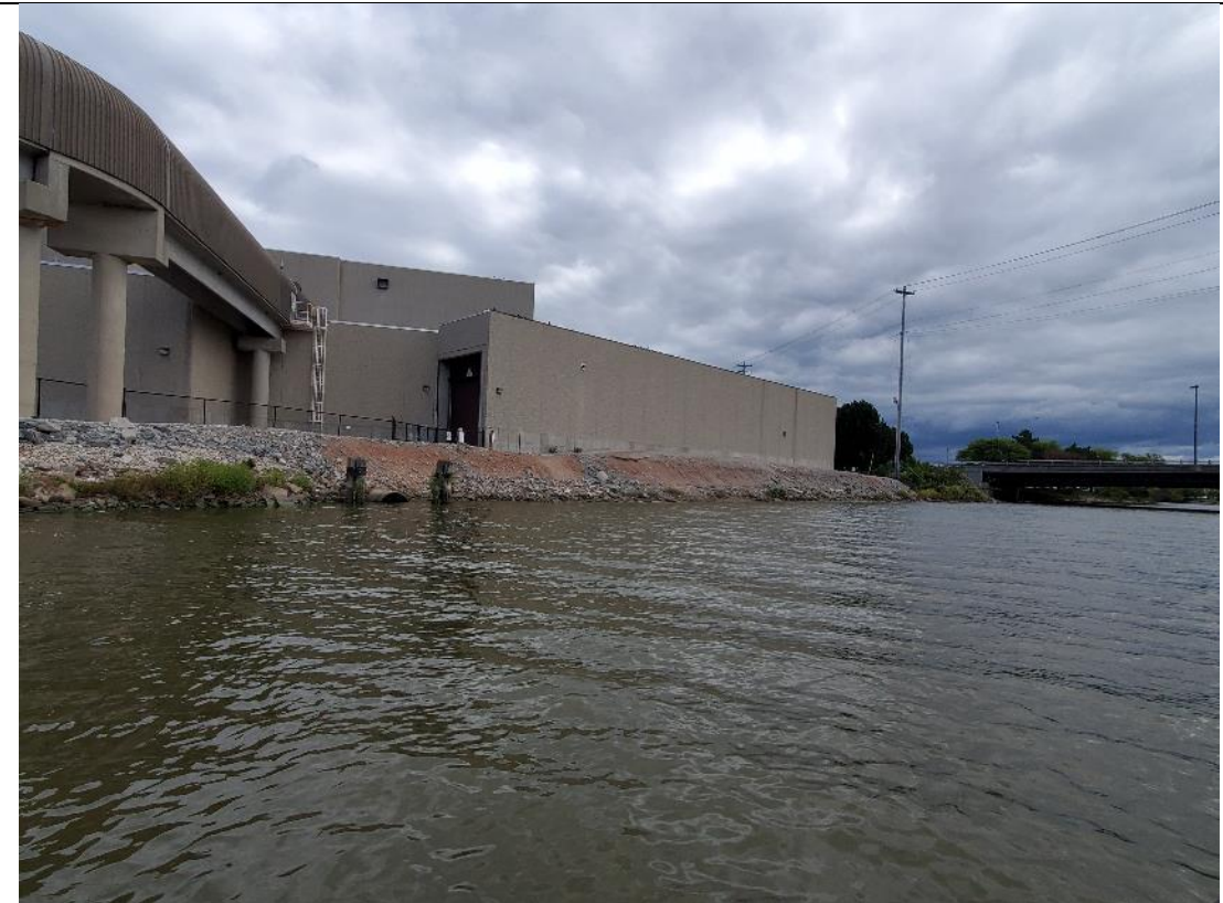
Eastern shore, approximate location of 12" line
