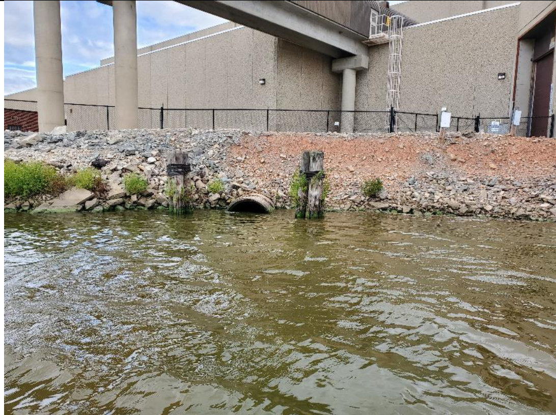
Eastern Shore, Culvert and possible cable location
