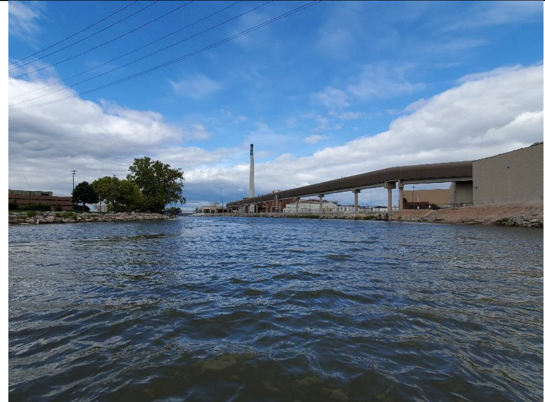
Downstream view (facing northwest)
