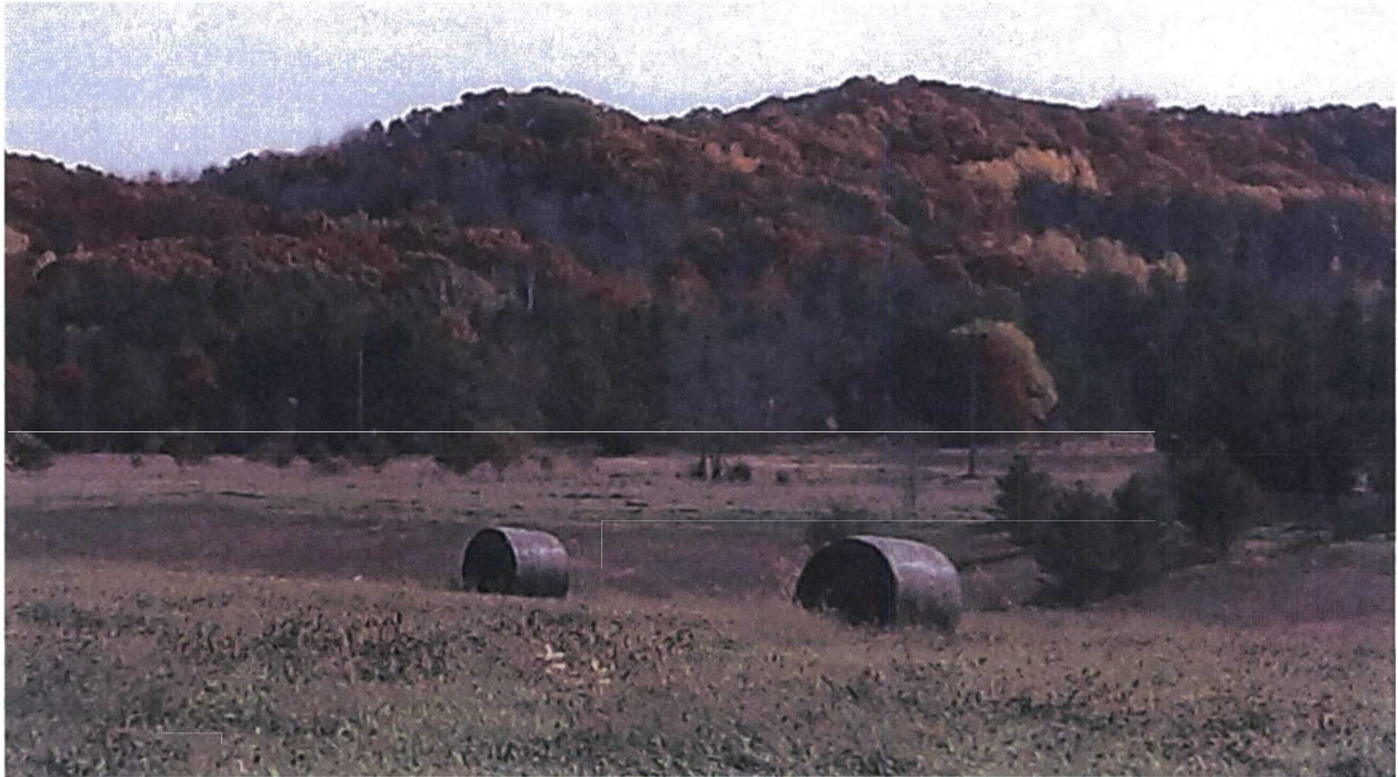
Melby Road Disposal Site Cap
