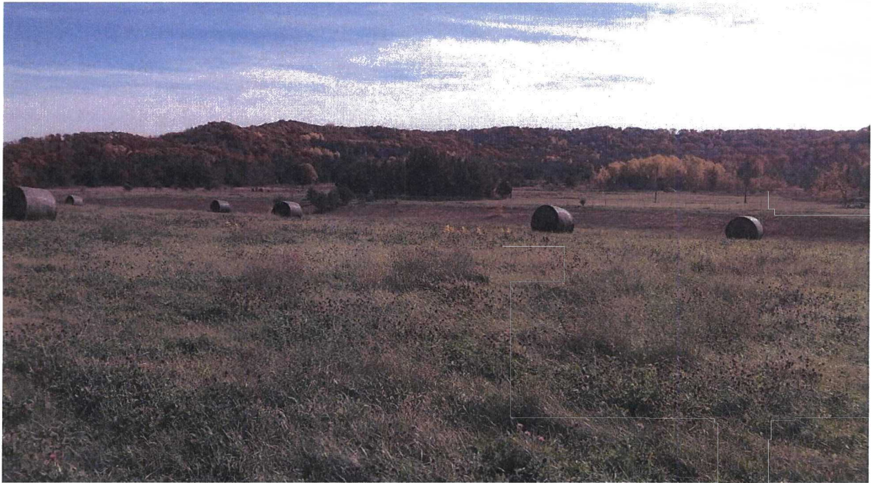
Melby Road Disposal Site Cap
