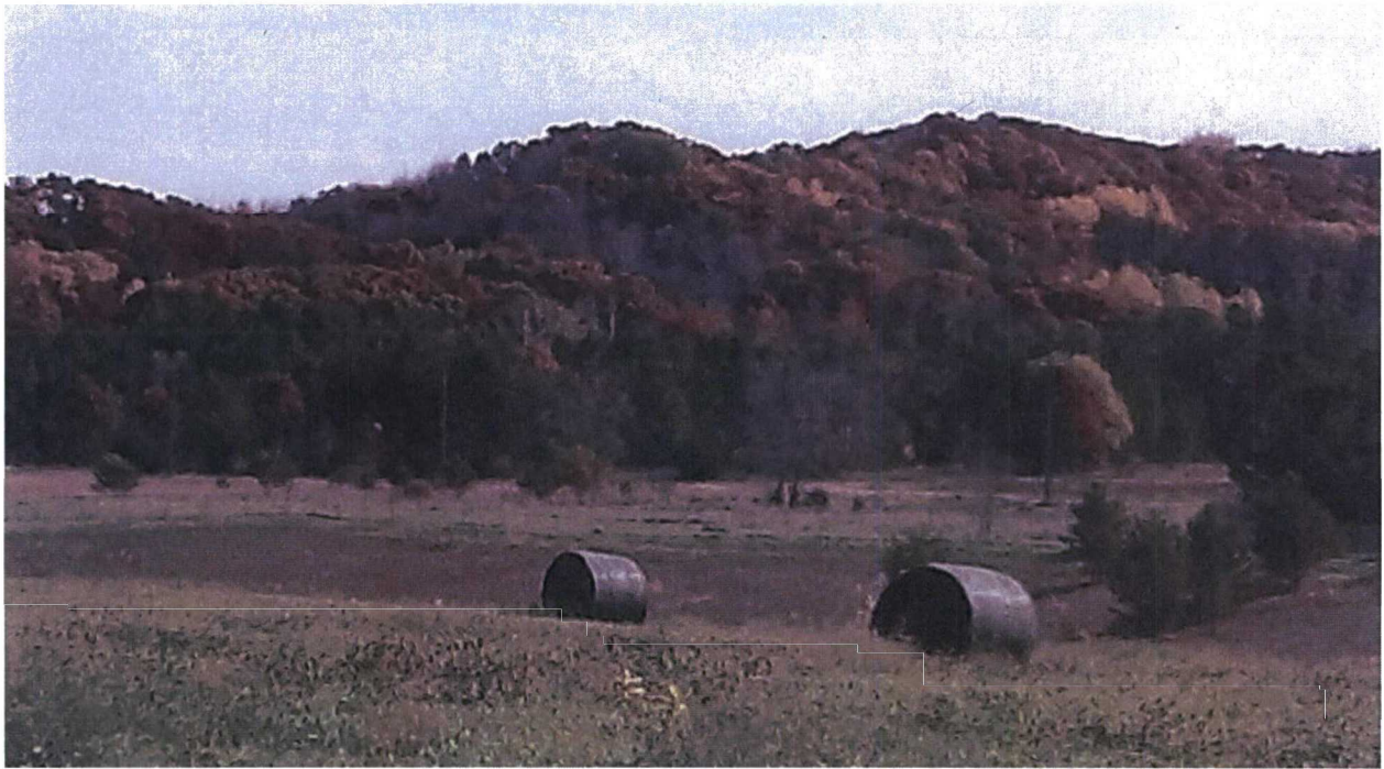
Melby Road Disposal Site Cap
