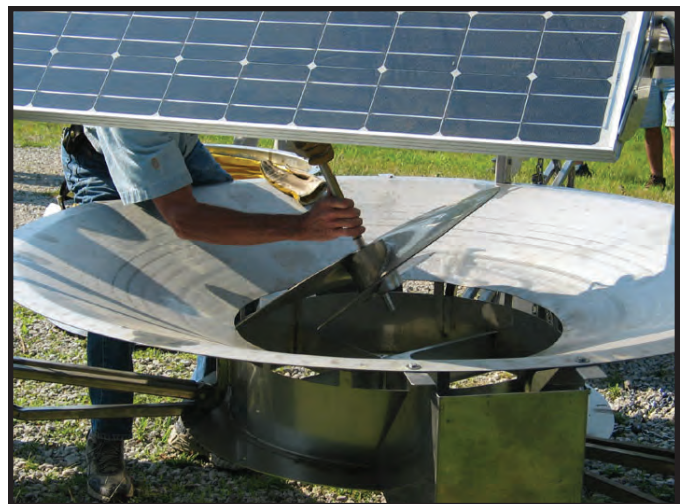
Impeller Removal For Buildup Below Impeller
