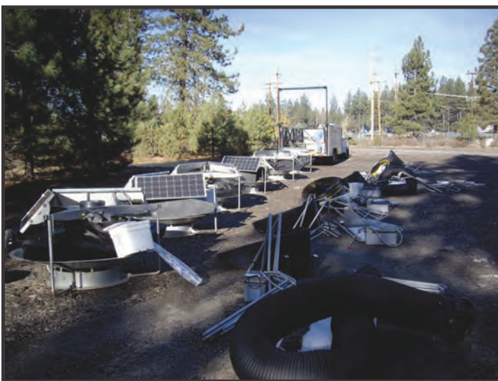
Staging Area With Disassembled SolarBee Units
