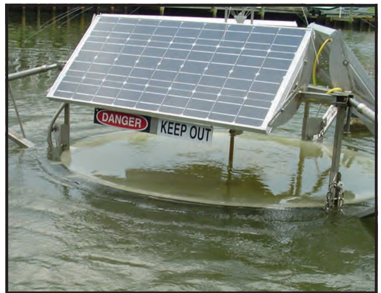
Flow Coming Off Distributor Dish
