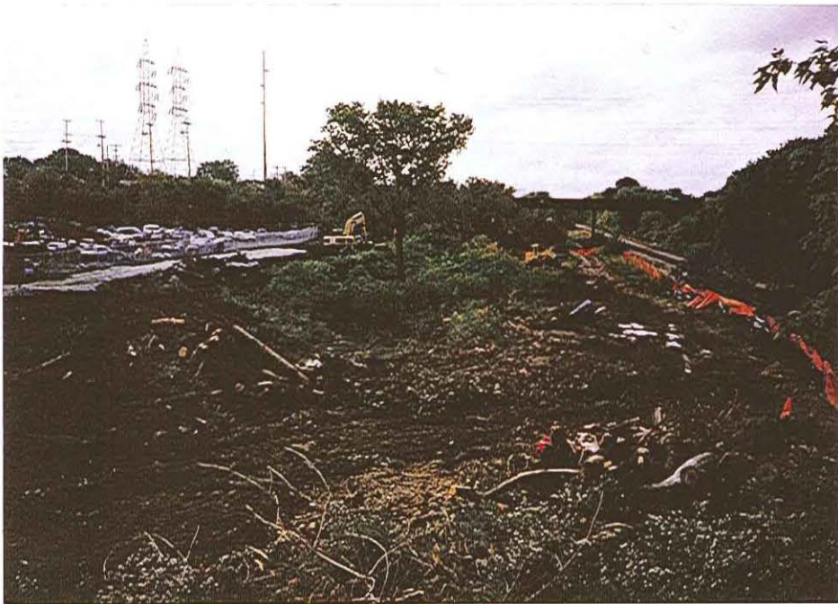
#3 - Site Preparation Work
