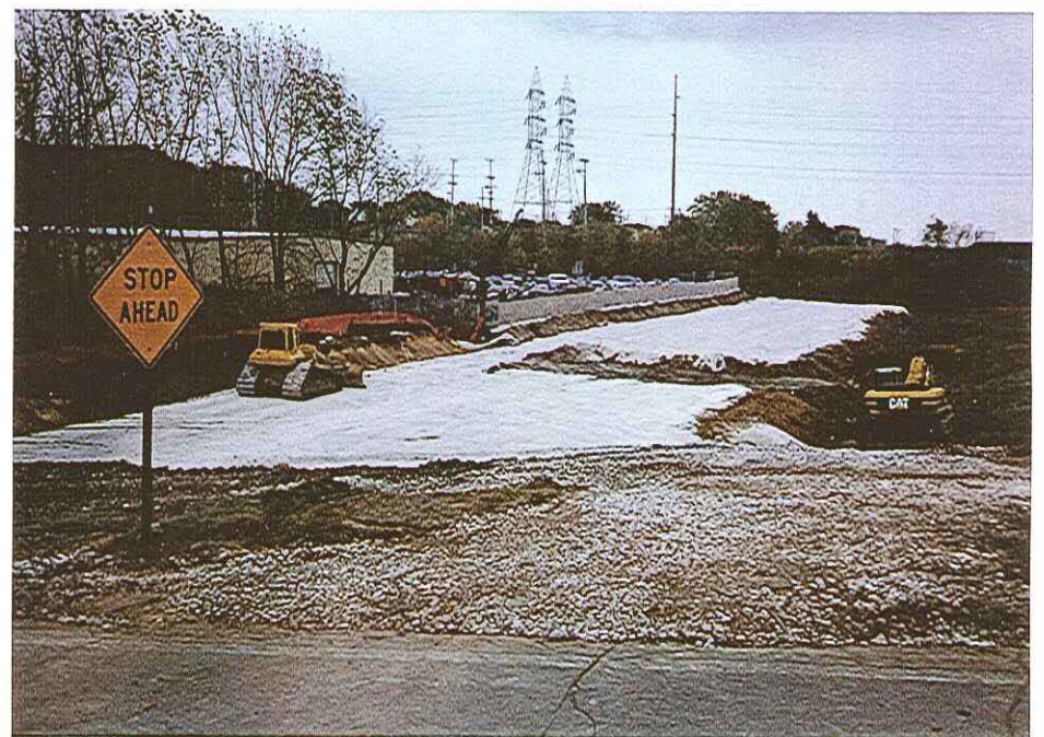
#20 - Barrier Placement Complete
