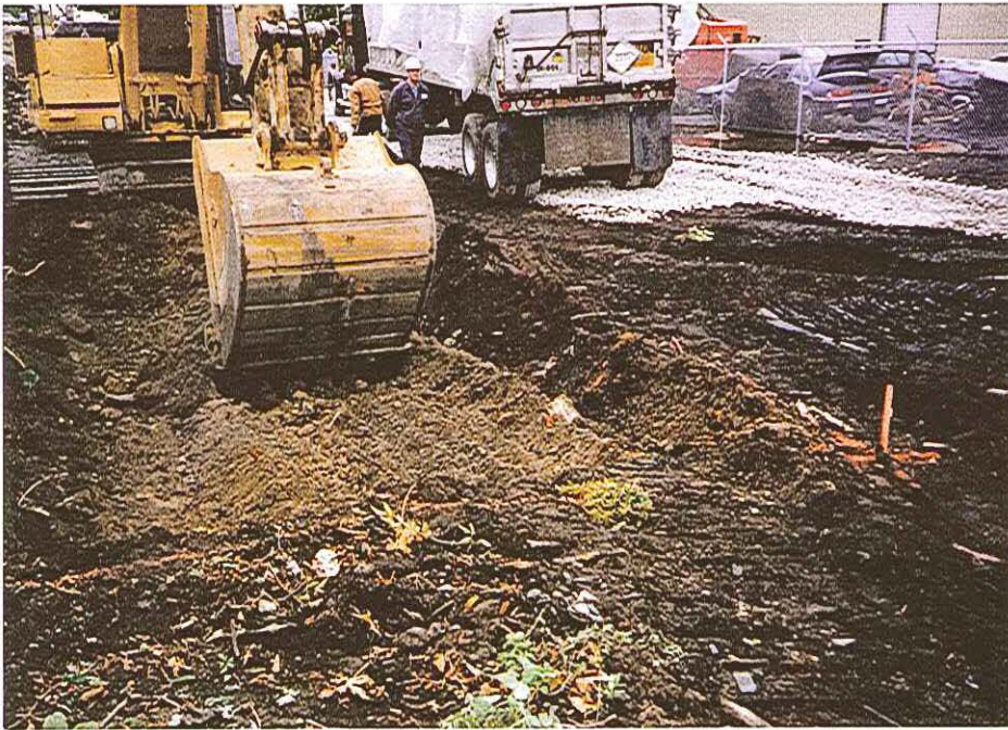
#5 - Excavating TSCA Waste
