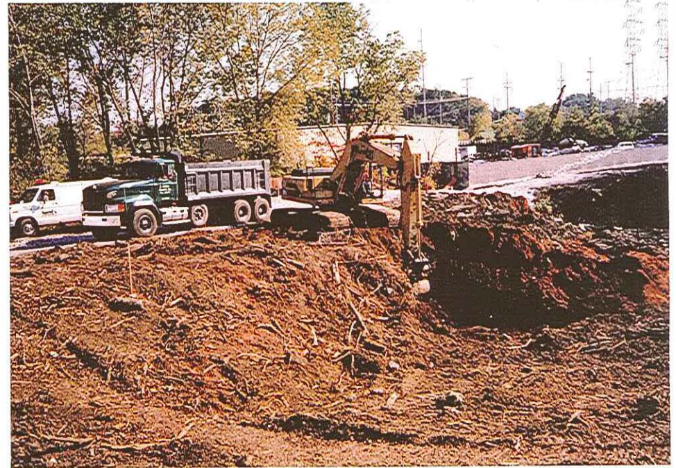
#8 - Loading Biopile Material
