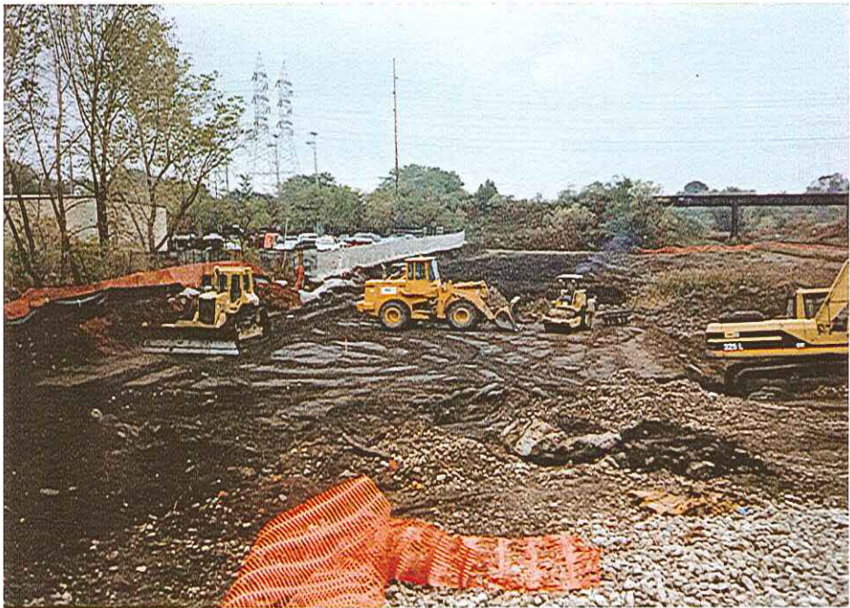
#15 - Grading and Compacting
