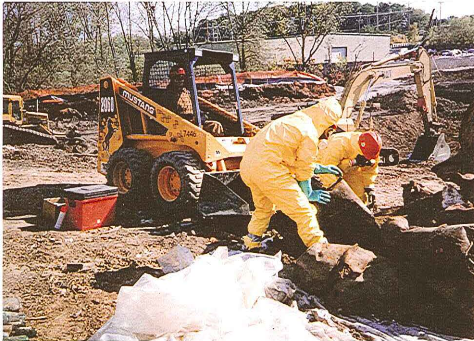
#11 - Drum segregation and characterization
