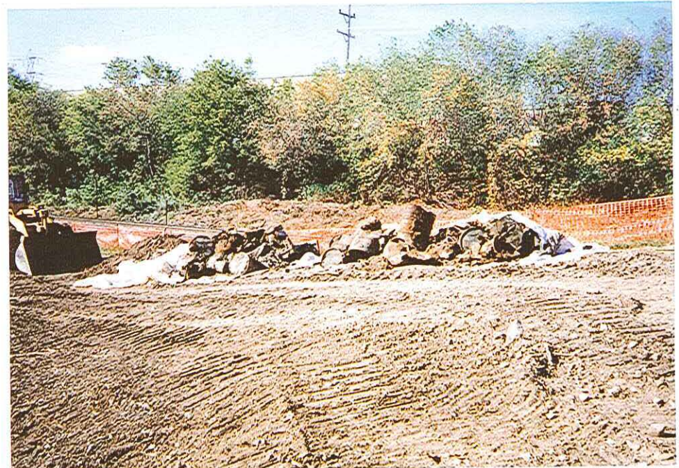
#12 - Drum segregation and characterization
