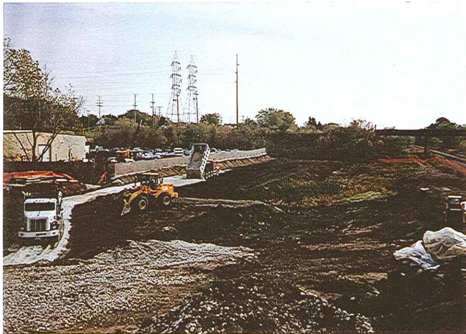
#19 - Placing Gravel Barrier
