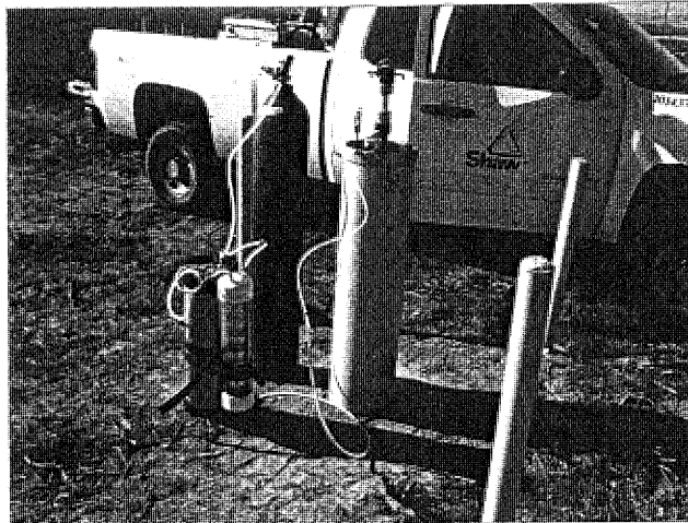
Exhibit 3. Nitrogen delivery system for the SDC-9™ bacteria injections
