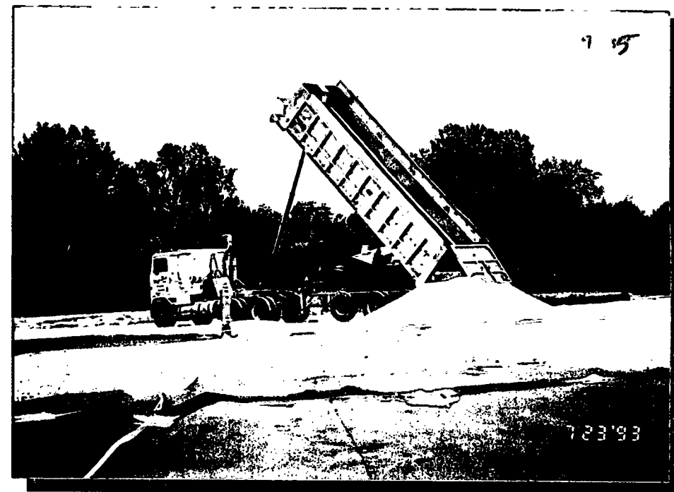
3. Placing working surface material over Type II geotextile.
