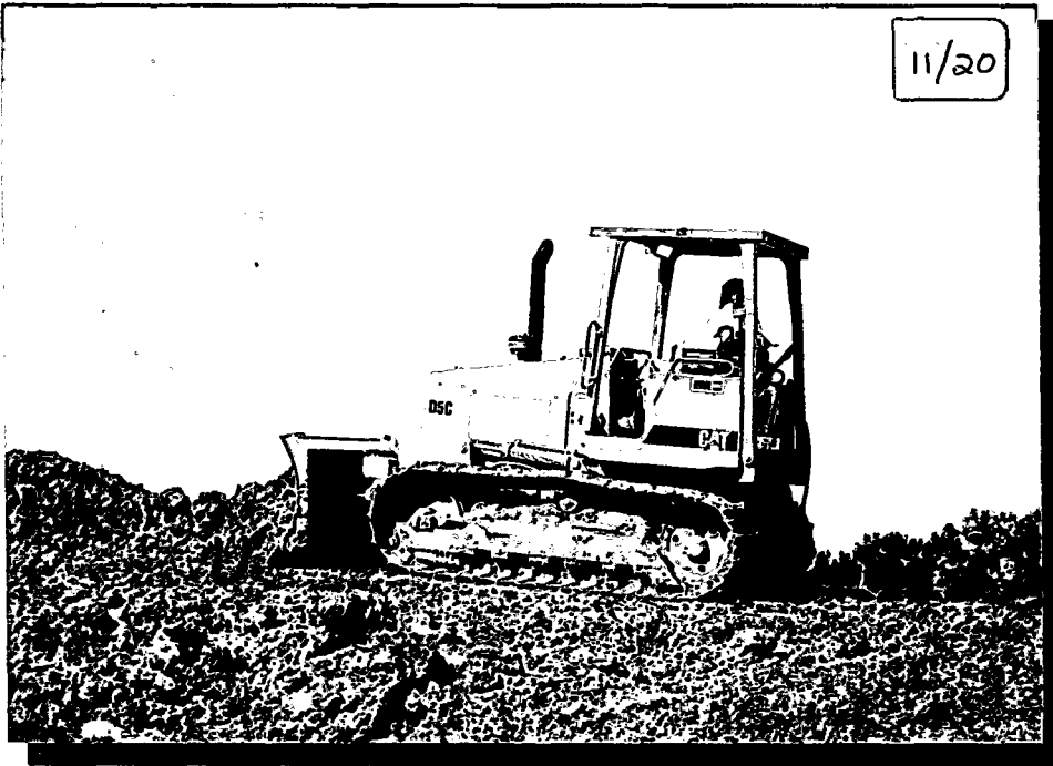
9. Cat DSC dozer working clay layer.
