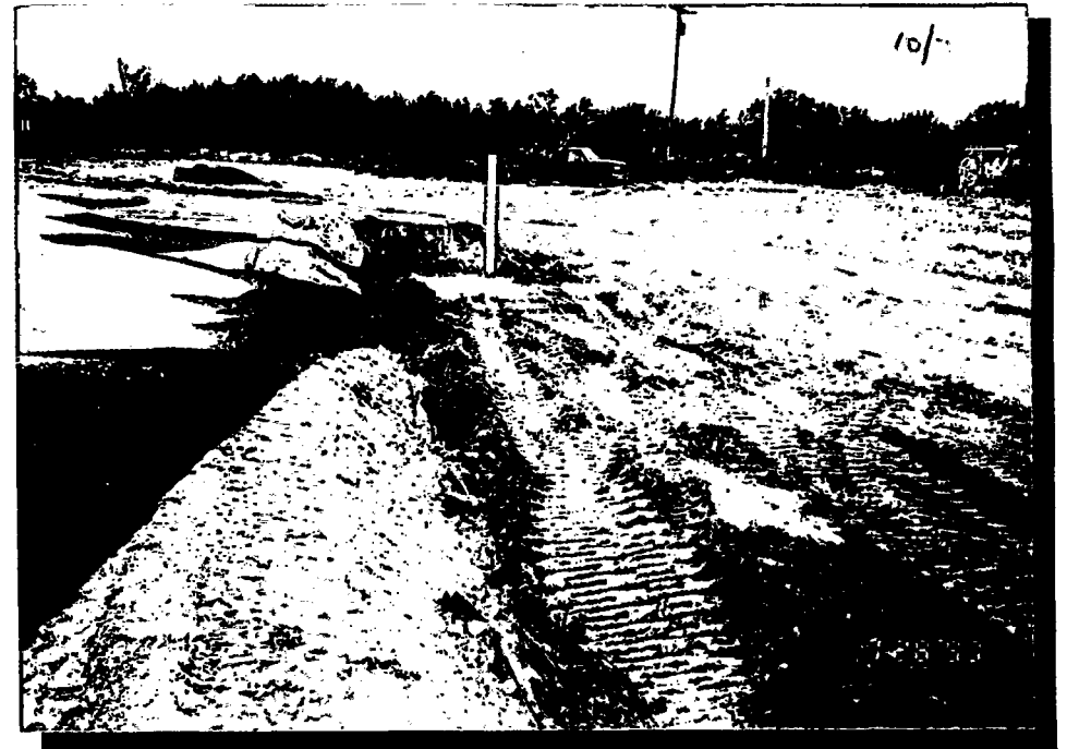
21. Construction of landfill gas interceptor trench.
