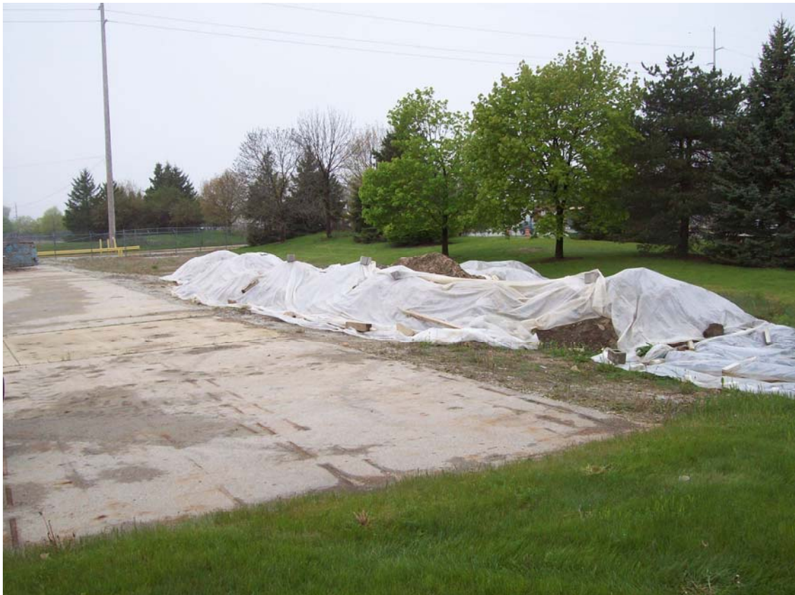
Photo 2 - Soil Pile Looking Northwest (prior to removal from site)
