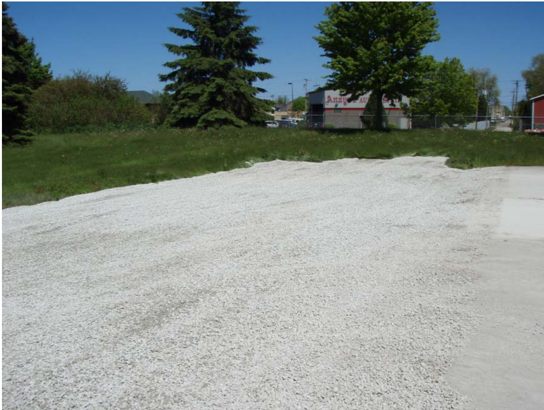
Photo 8 - Soil Pile Area Looking Northeast (after final backfilling)
