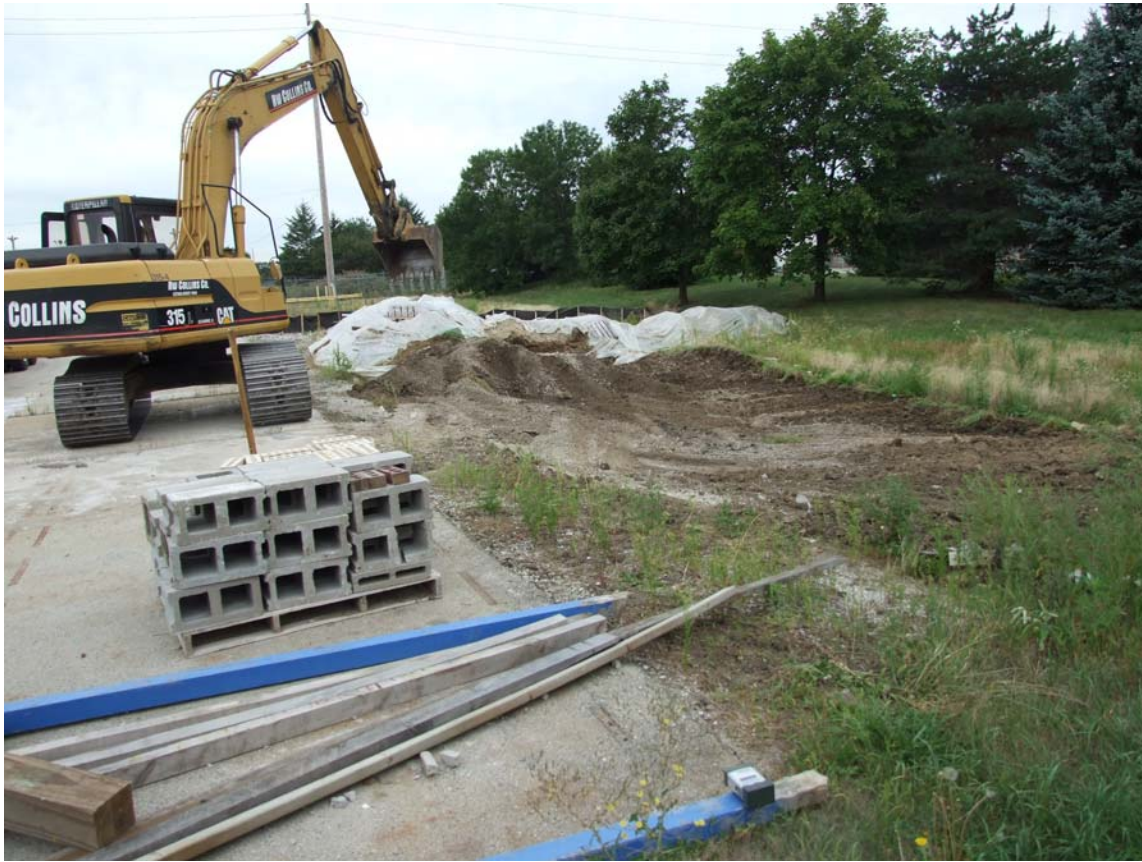
Photo 3 – Soil Pile Looking Northwest (during removal from site)
