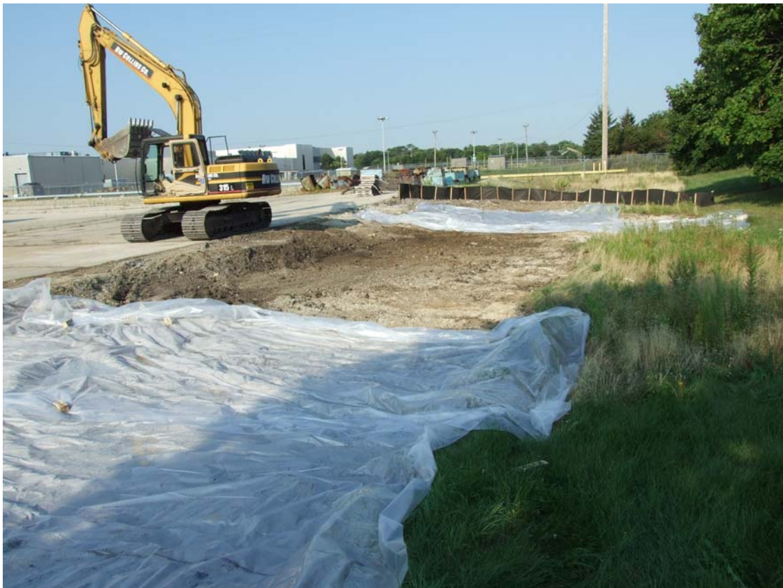
Photo 4 – Soil Pile Looking Southwest (after removal from site)
