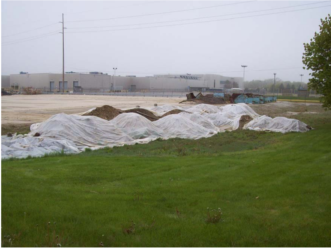
Photo 1 - Soil Pile Looking Southwest (prior to removal from site)
