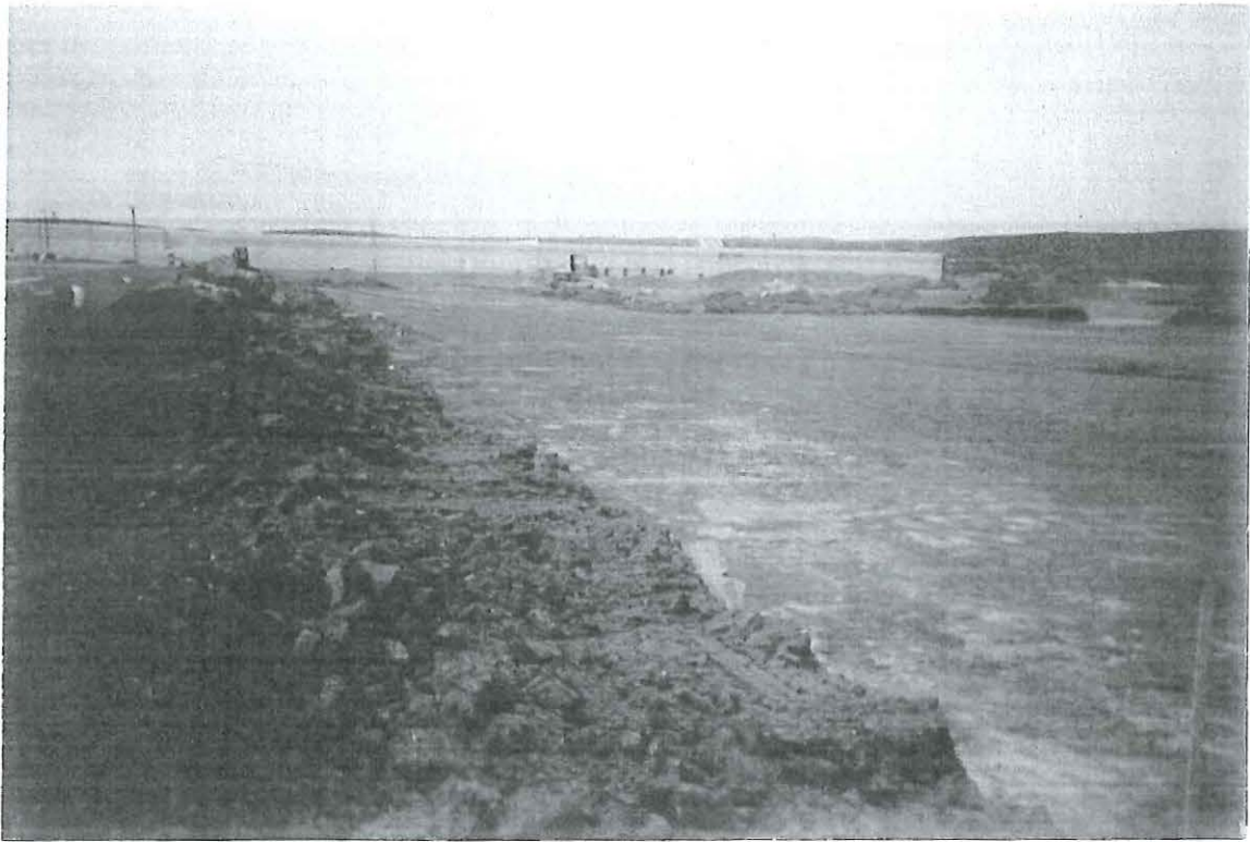
Photograph shows the completed excavation: southeast corner of Area 24, looking west.
