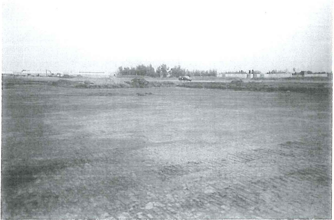
Photograph shows the completed excavation: northwest corner of Area 18, looking southeast.
