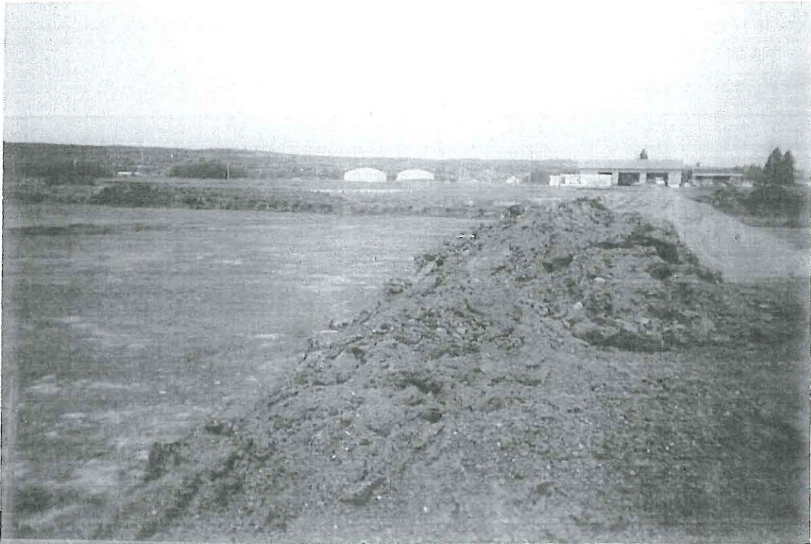
Photograph shows the completed excavation: southeast corner of Area 24, looking north.
