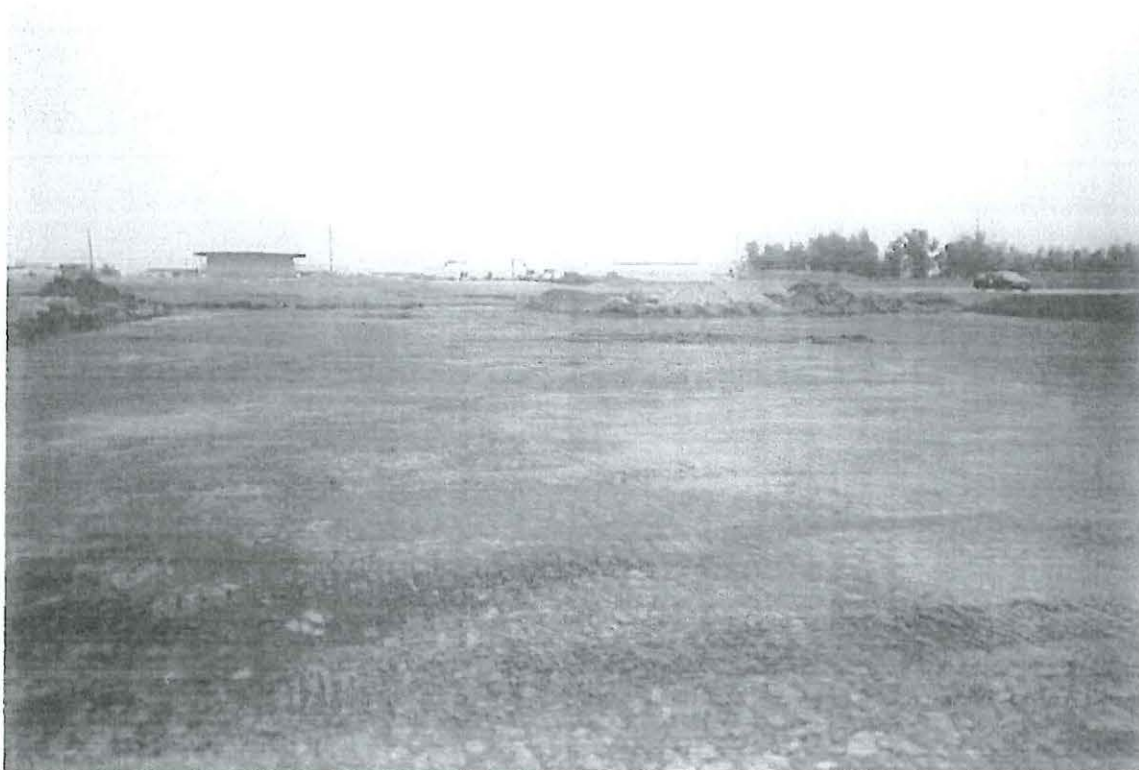
Photograph shows the completed excavation: northwest corner of Area 18, looking east.
