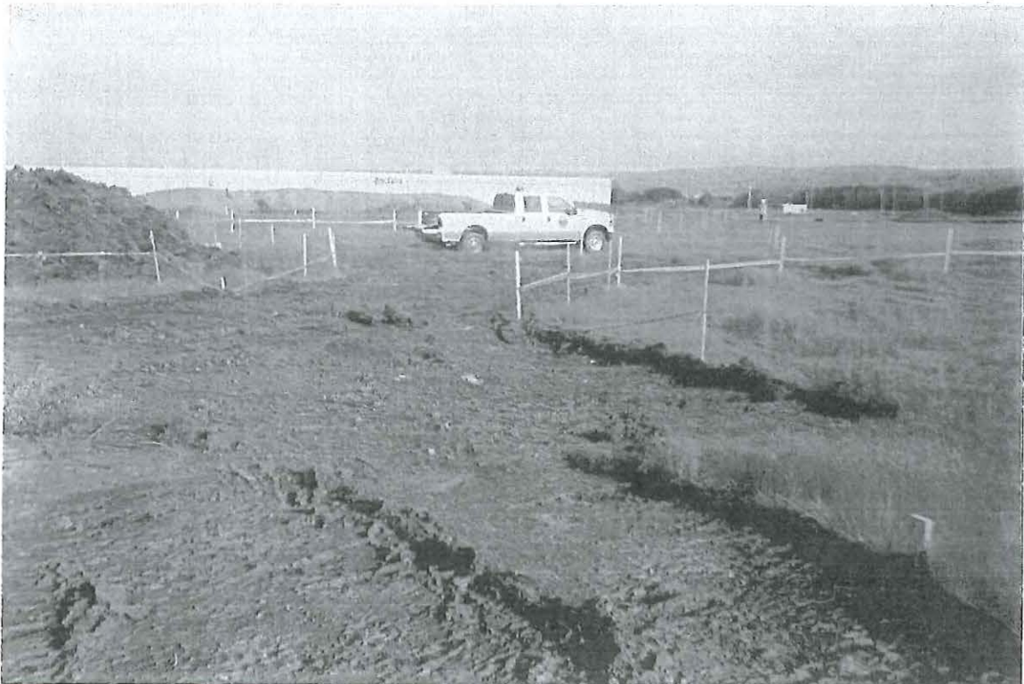
Photograph shows sod stockpiled outside of the excavation boundary.
