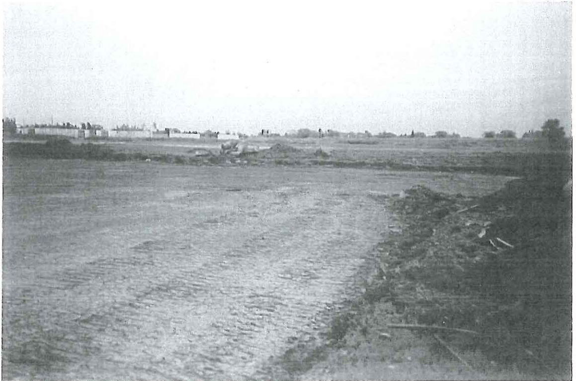
Photograph shows the completed excavation: northeast corner of Area 18, looking south.
