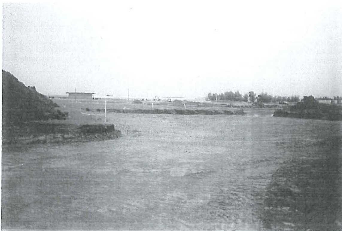
Photograph shows the completed excavation: southeast corner of Area 6, looking southeast.
